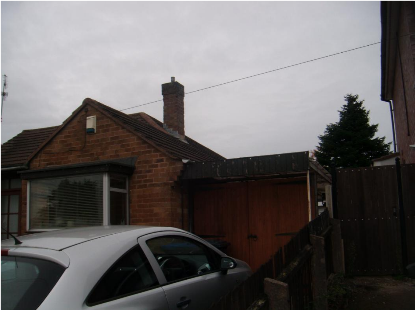
Side: intact tiles and single storey garage (no loftspace/plastic clear roofing)
