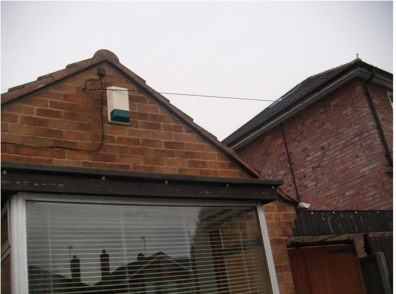
Front gable detail: intact
