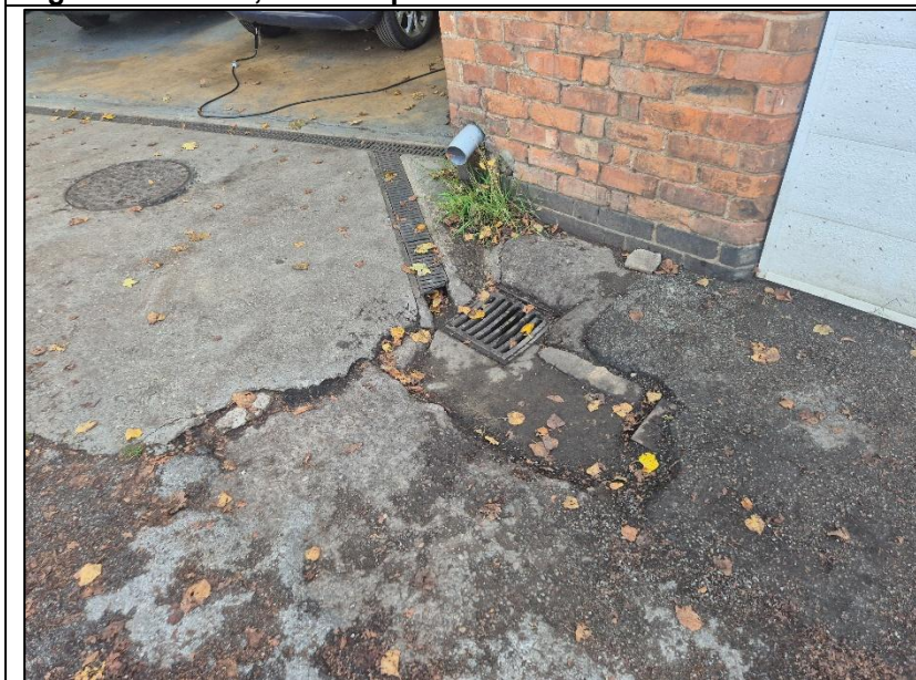
Figure 9. Slit drain and associated gulley pot.
