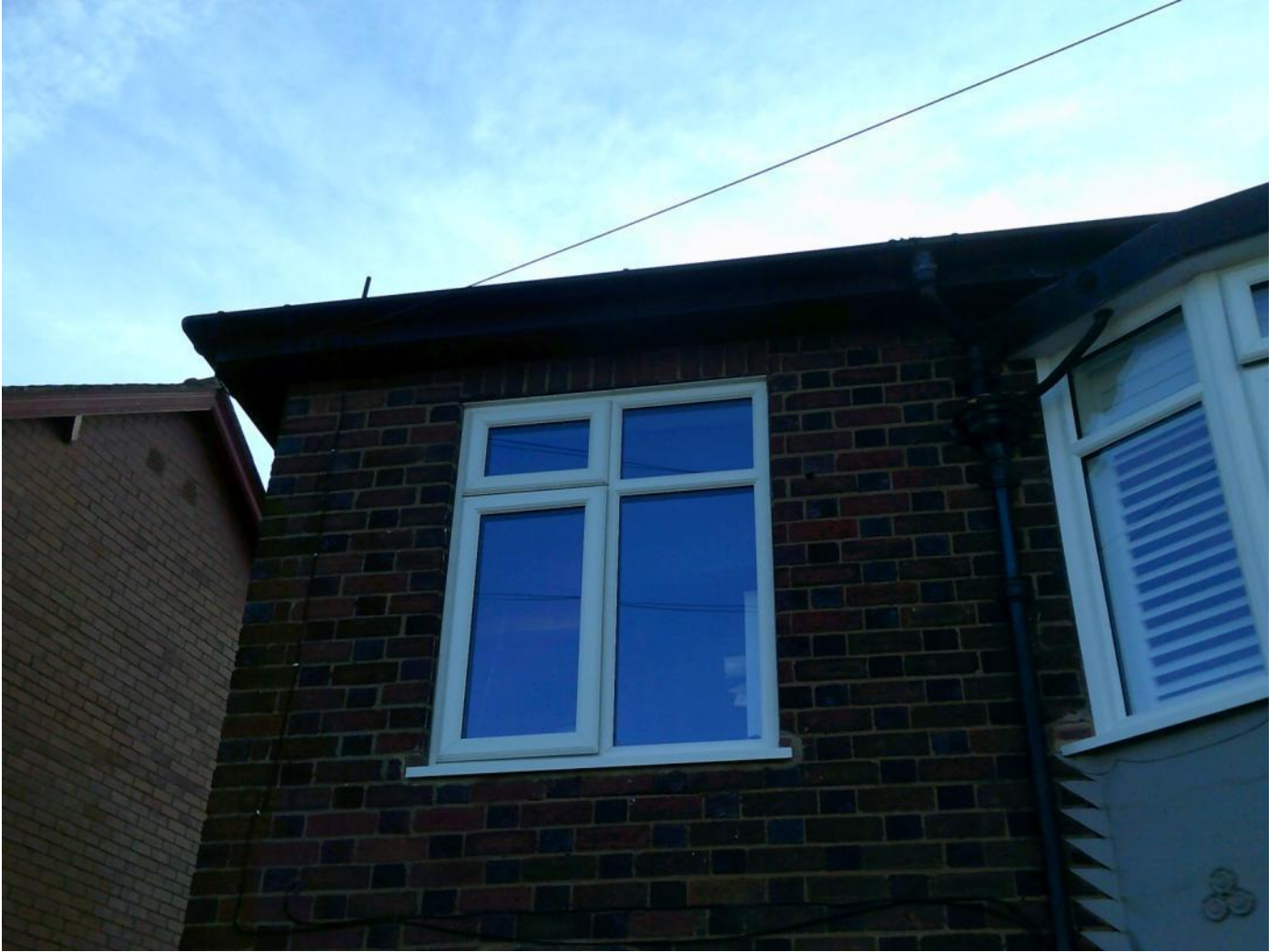
Front intact soffits and bay
