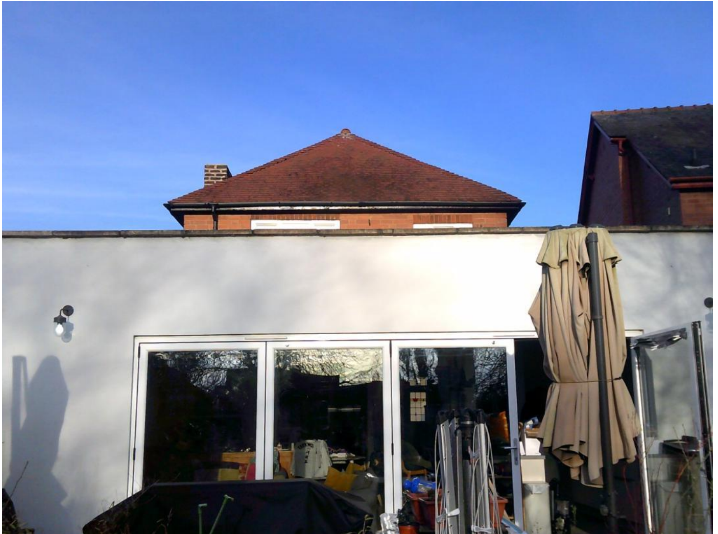
Rear extension and main house behind
