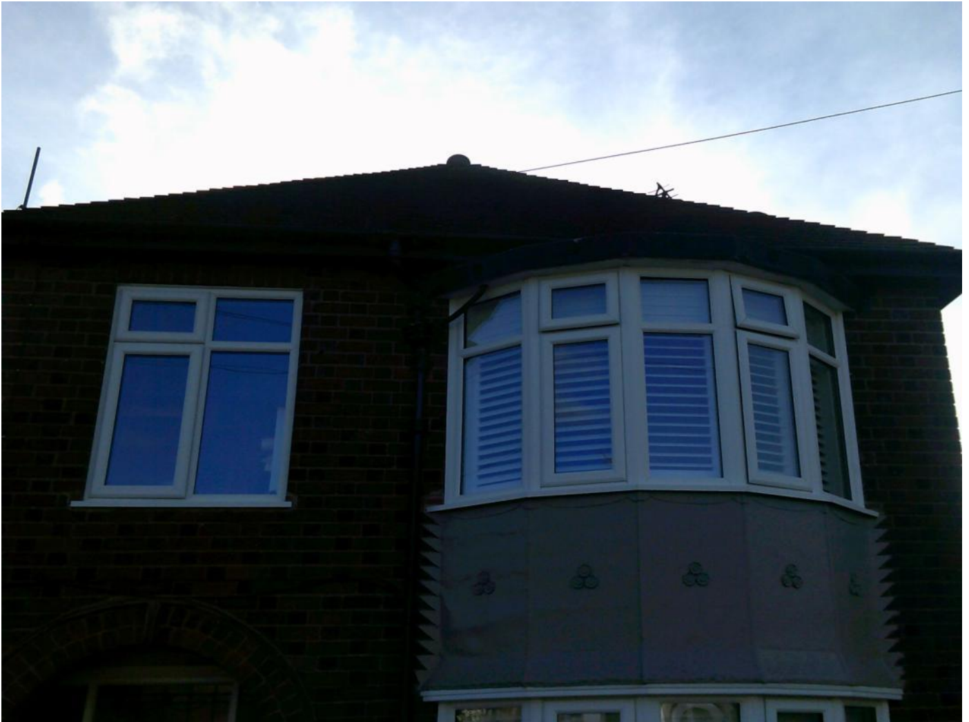
Front bay/roof intact
