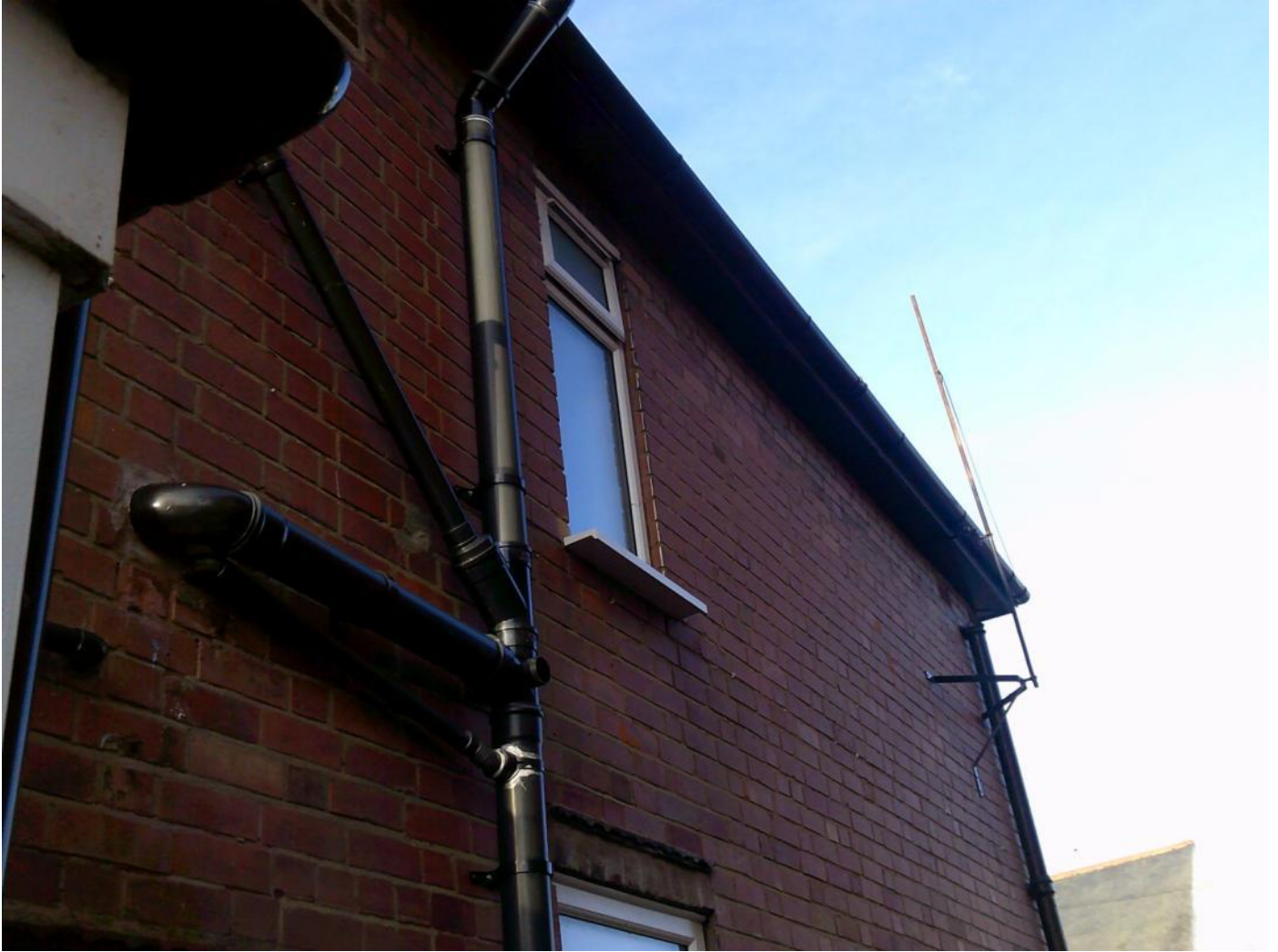
Side elevation soffits intact
