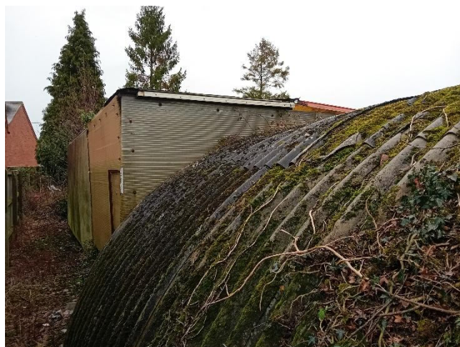
Photo 10: South and east elevations of building B2a.
