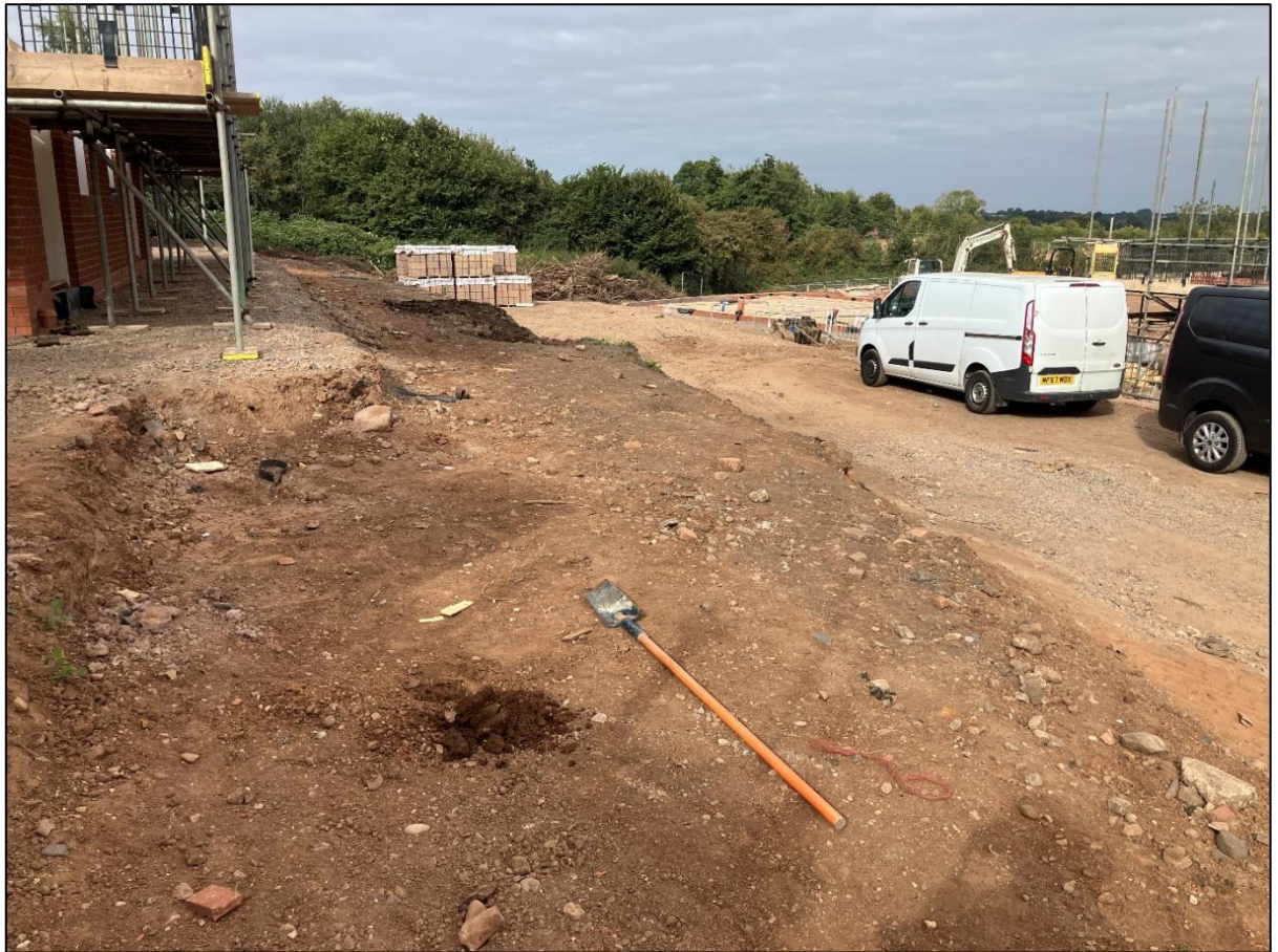
Figure 3-B: Soil within the vicinity of SL01
