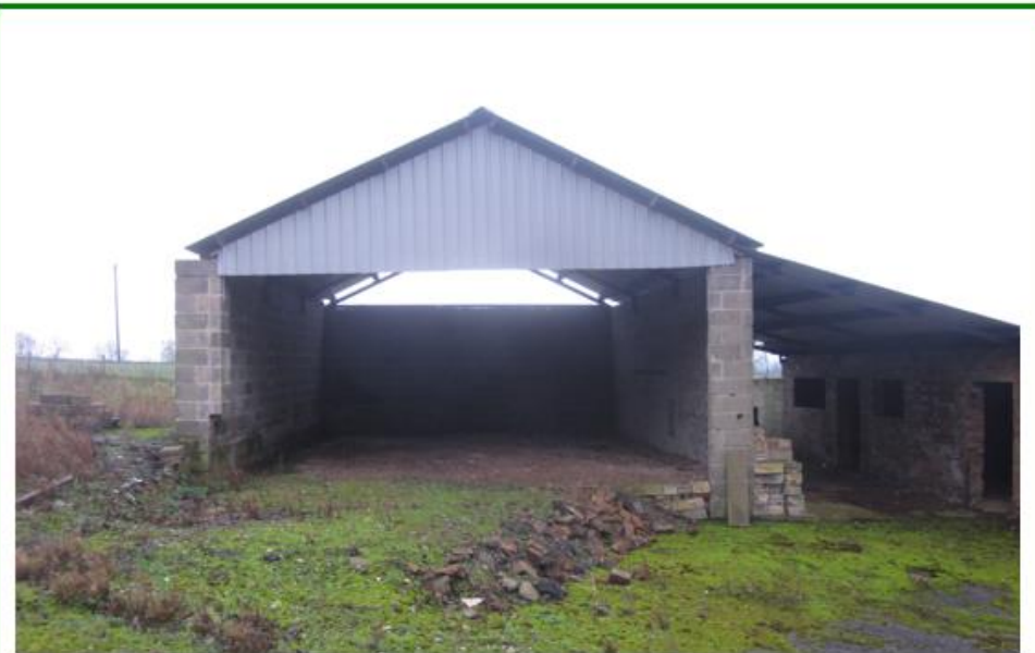
Photo No.14: Facing SE showing Barn No.4, the north eastern most barn on site and infilled with made ground base
