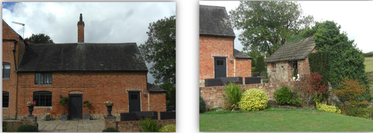
Fig .12 & 13 Old Hayes Farm - Existing views from the garden.
