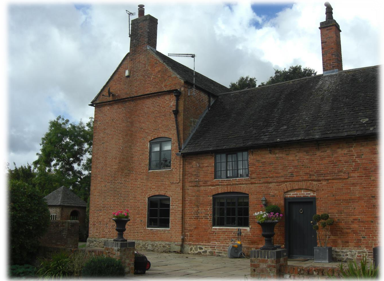
Fig .11 Old Hayes Farm showing the connection between the two and three storey elements.
