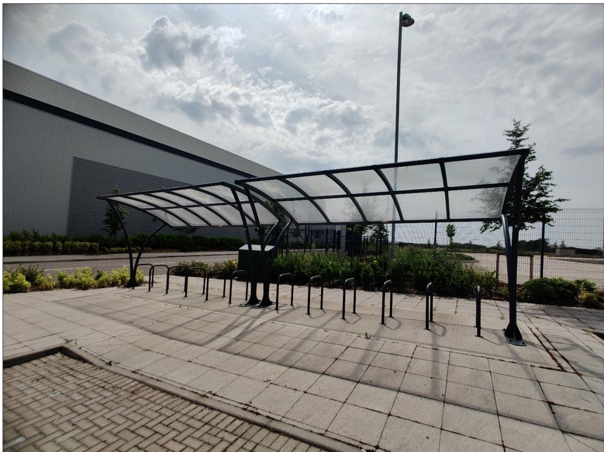
Figure 2.1: Sheffield Stands at Building Entrance
