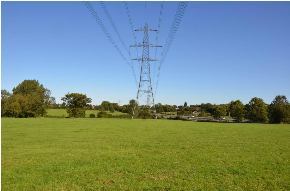
Figure 13. Field J, view to southeast, towards adjacent M69 motorway
