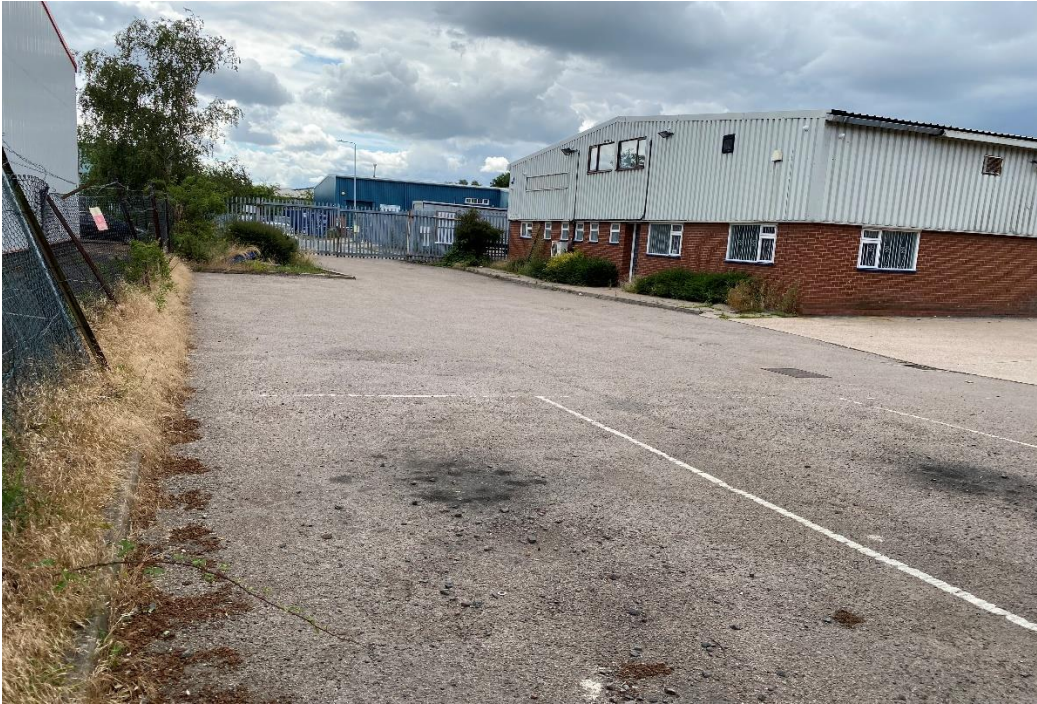
Photo C: Taken from Hardstanding position C (site of visitor parking and front entrance to building)
