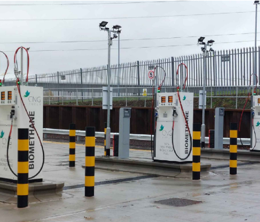
TYPICAL PUMP ARRANGEMENT ALL FLOODLIGHTS ON PUMP ISLANDS TO BE ONE AT 10° AND ONE AT 30° ELEVATION.
