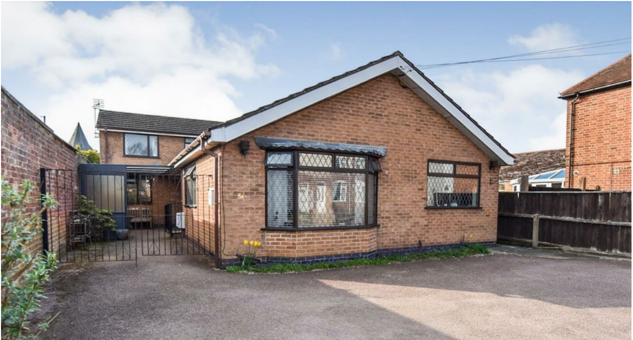
Photograph 1 – Front Driveway and Parking
