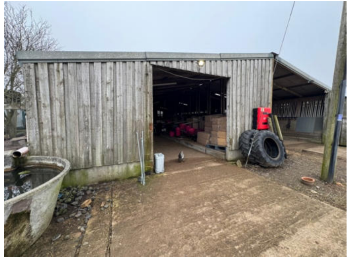
Photo 2: Building B1 exterior
