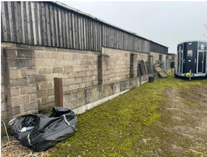
Photo 9: Building B2 external
