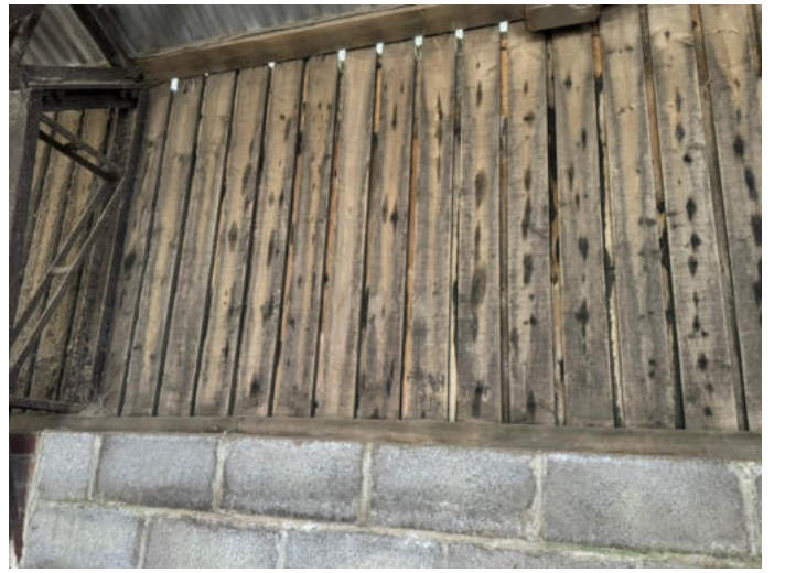
Photo 10: Building B2 interior
