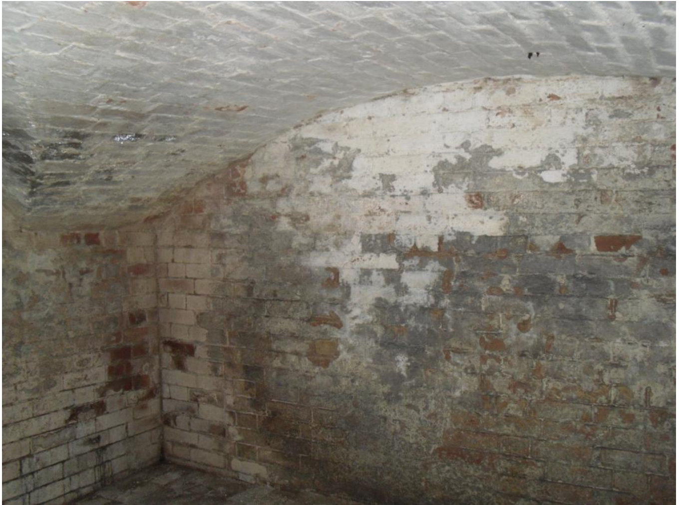
Cellar to building 1
