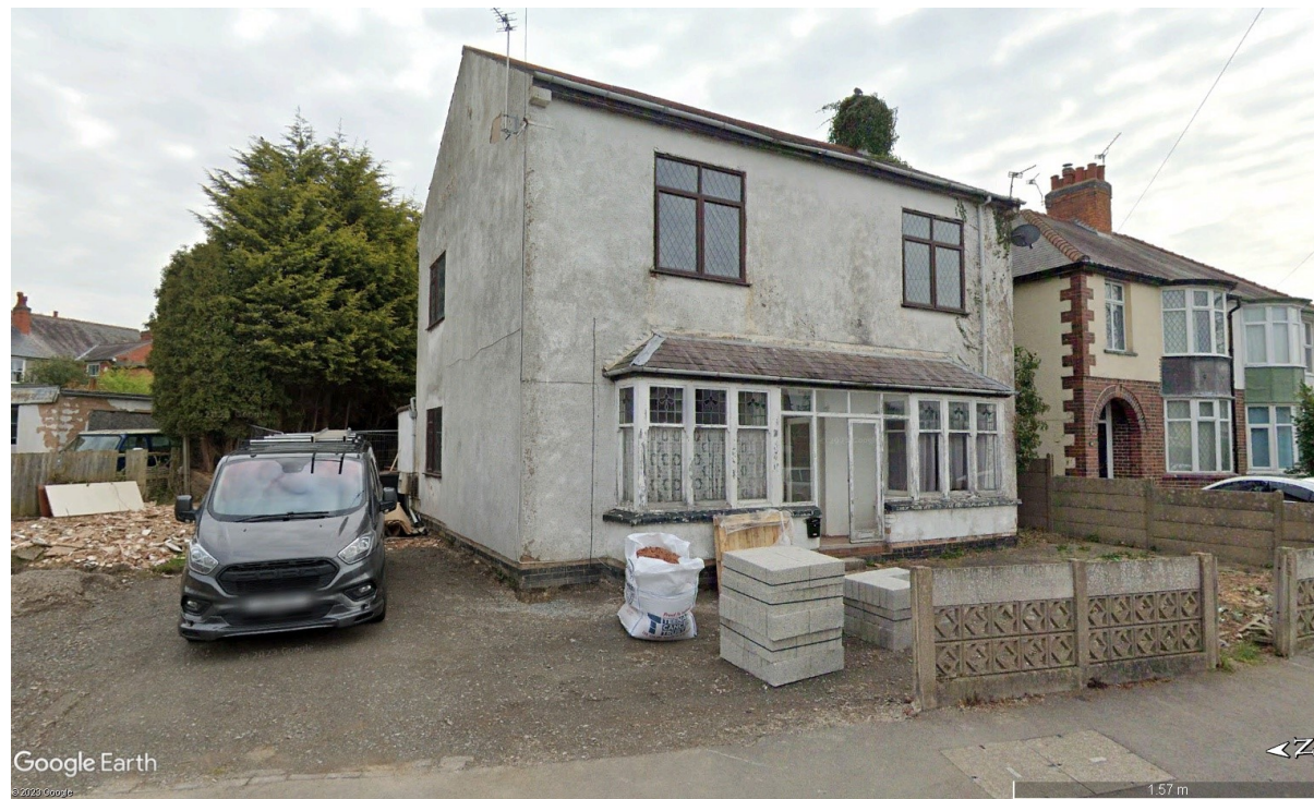
No.40, currently undergoing refurbishment.
