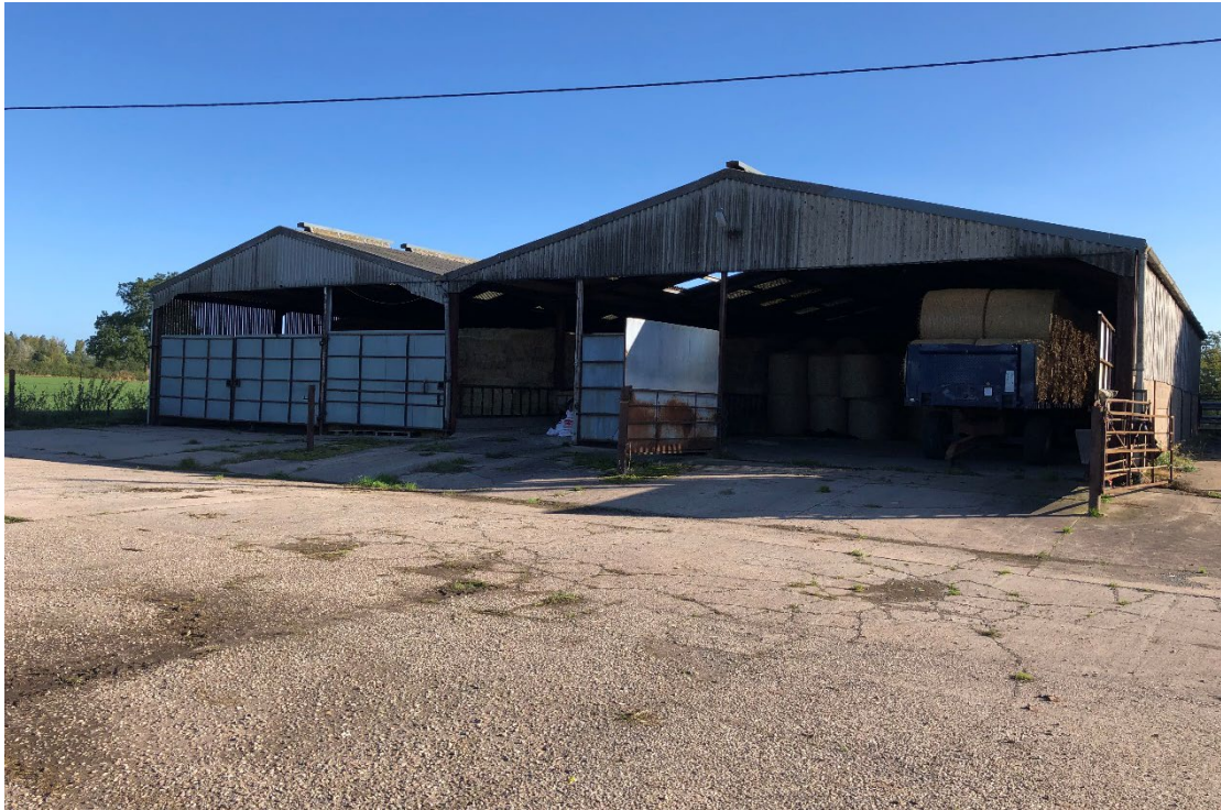
[The west elevation of agricultural building 1 together with adjacent hardstanding. Photograph taken on 21 st October 2021]
