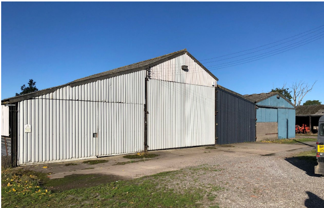
[The east elevation of agricultural building 2 together with adjacent hardstanding. Photograph taken on 21 st October 2021]
