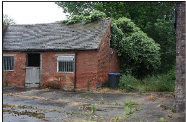
Figure 19. Hard Standing around Farm Buildings
