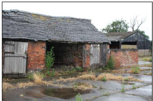
Figure 21. Hard Standing around Farm Buildings
