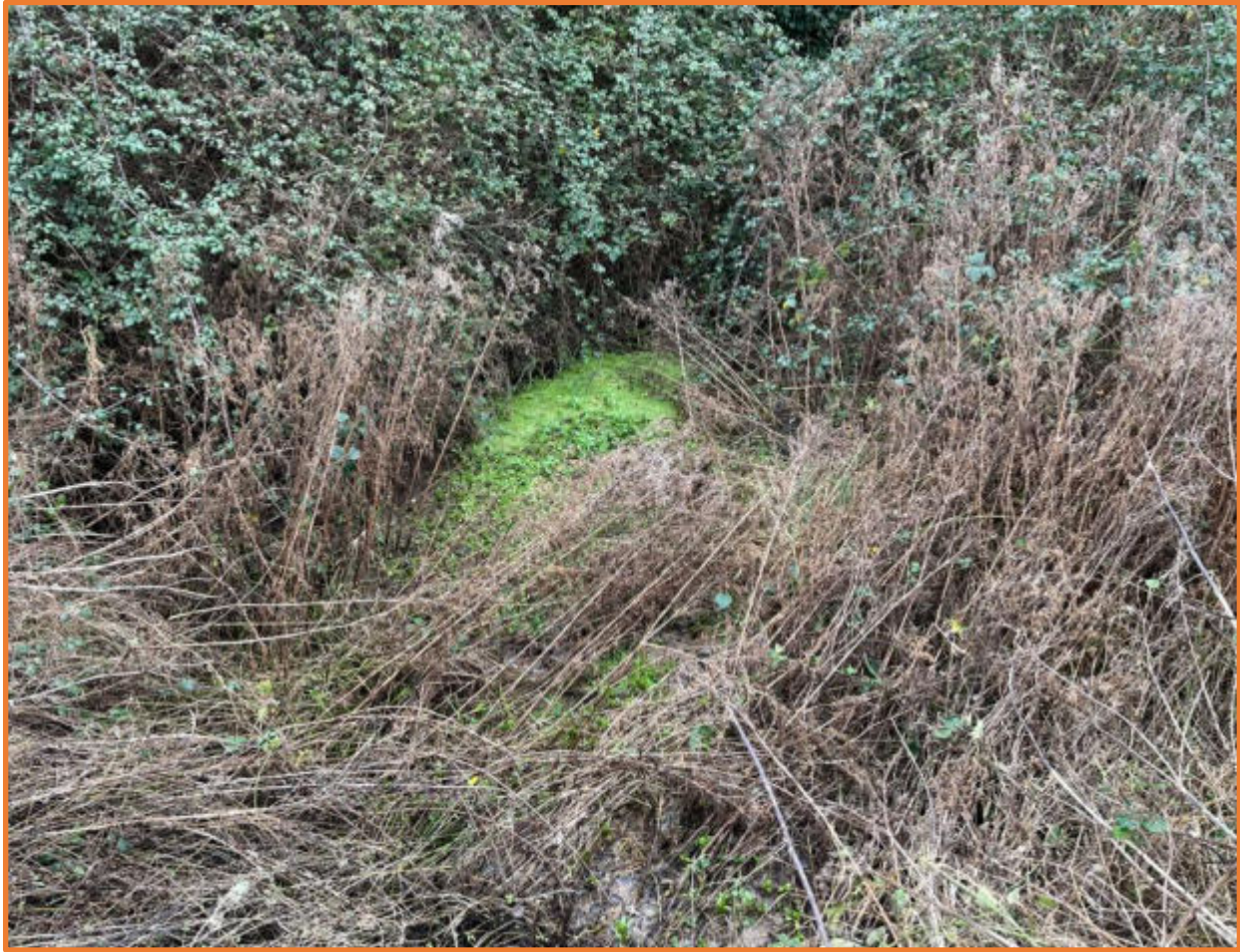
Figure 6: Outfall ditch; Northern parcel southern catchment.
