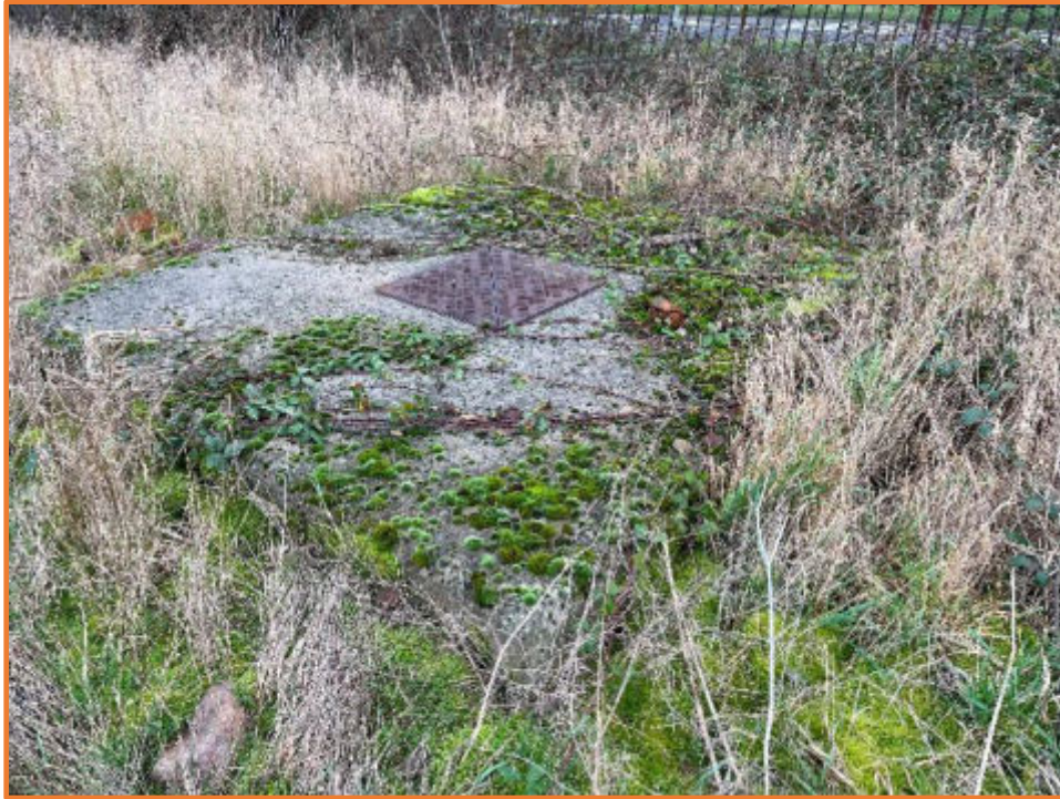
Photo of manhole 1602 on the combined sewer in the field to the north of the site.
