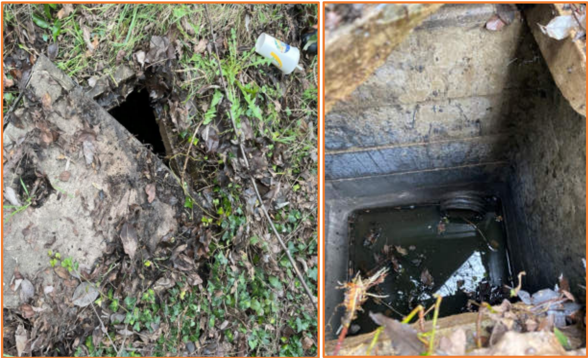
Figures 3a/b: Photo of the upstream manhole chamber on the piped surface water drain (left), and a view inside the manhole chamber (right).
