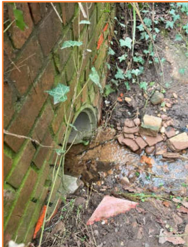
Photo of culvert beneath Rogue's Lane in the far north-west corner of the site.
