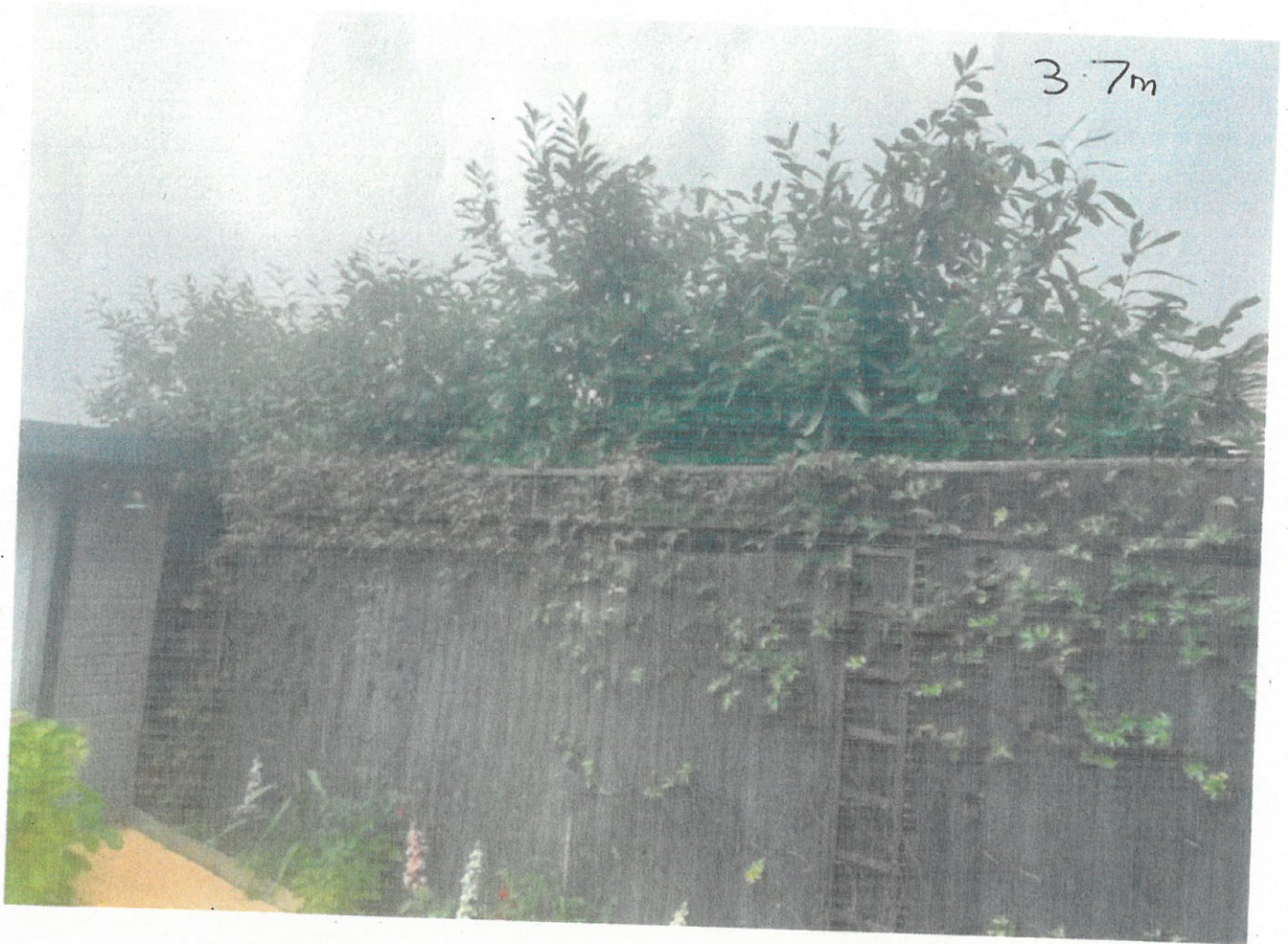
ANNEX E - SHOWS HEIGHT OF TREES AT THE HIGHEST POINT (DEC 2024)
