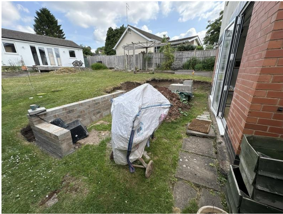
Construction of a patio to left hand side
