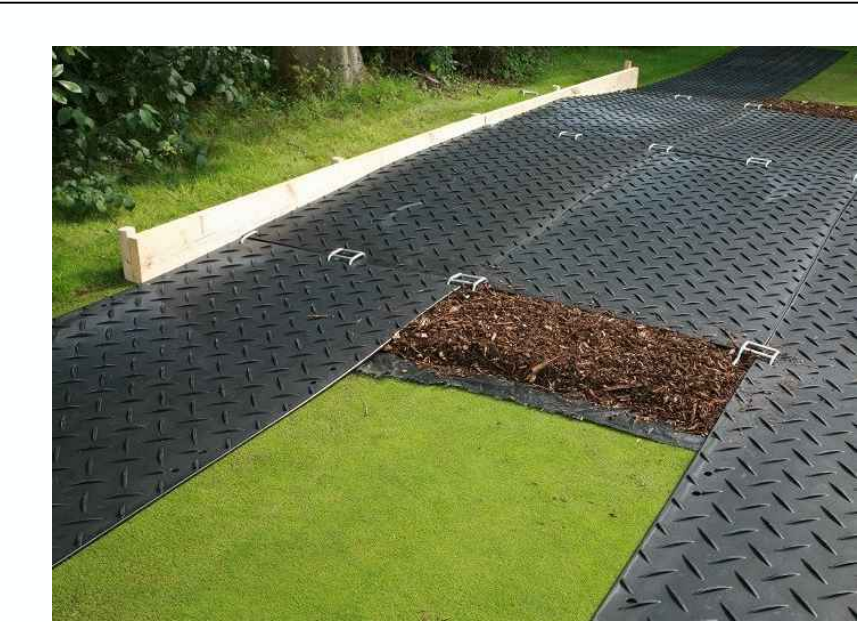
EXAMPLE: GroundGuards temporary ground protection
