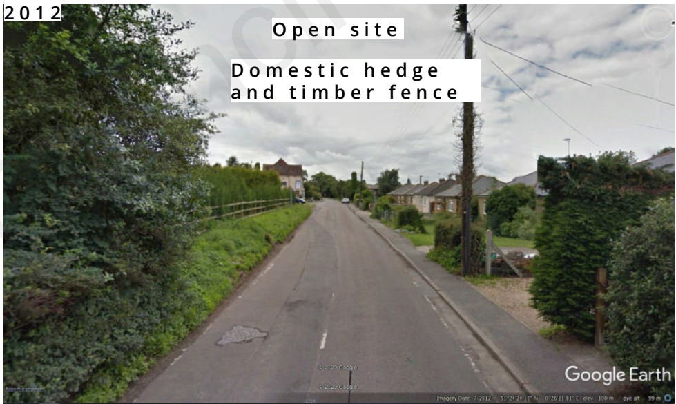
Image 4 - Google Earth Street View - 2012
