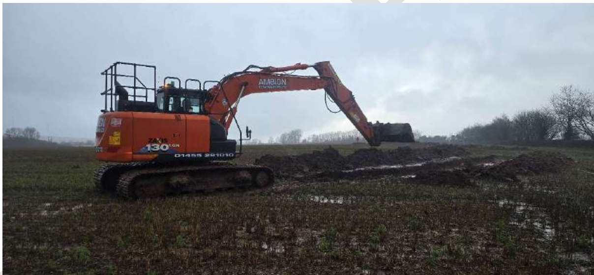
Figure 3: machining in progress; view west
