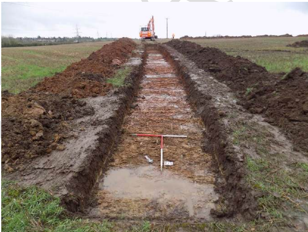
Trench 10: view south-west
