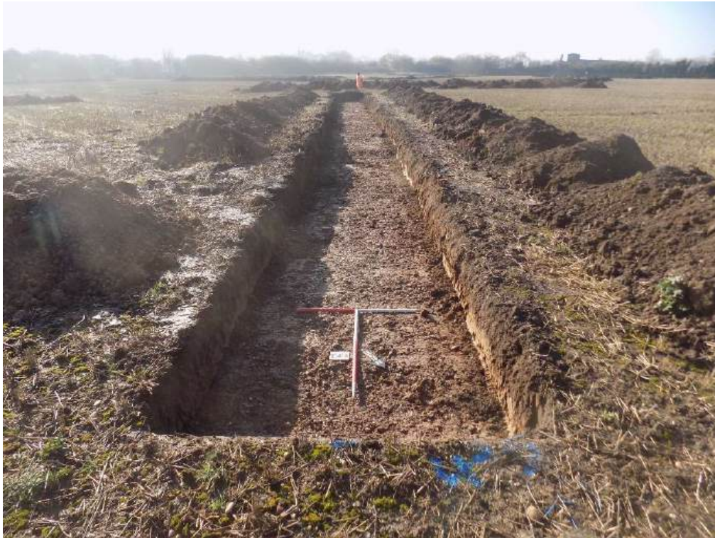
Trench 43: view south-west
