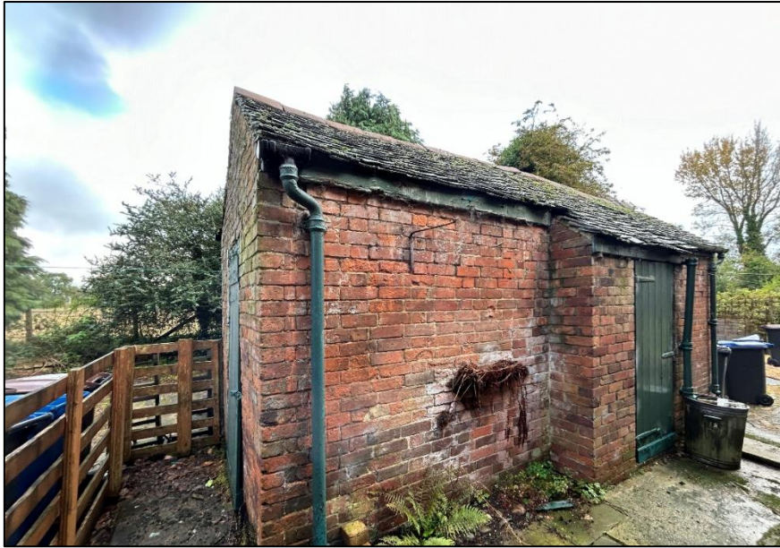
Plate 2. Outbuilding to be demolished
