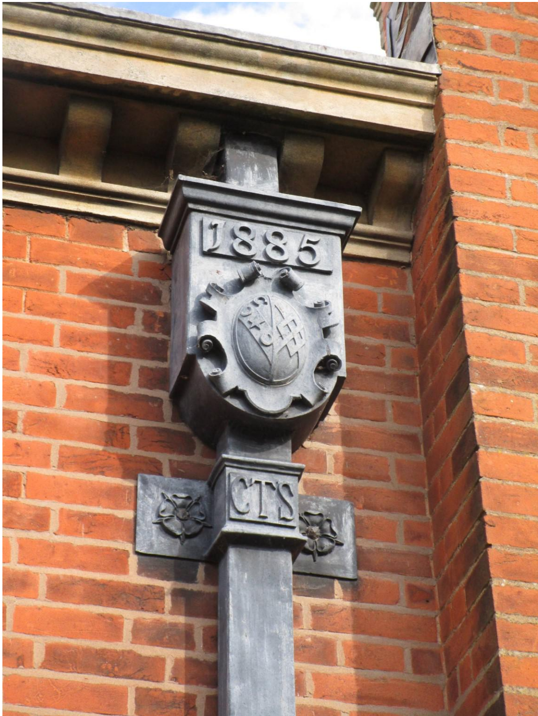
Plate 6: View of hopper and rainwater pipe detail.
