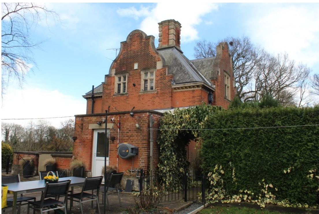
Plate 4: View from northwest.
