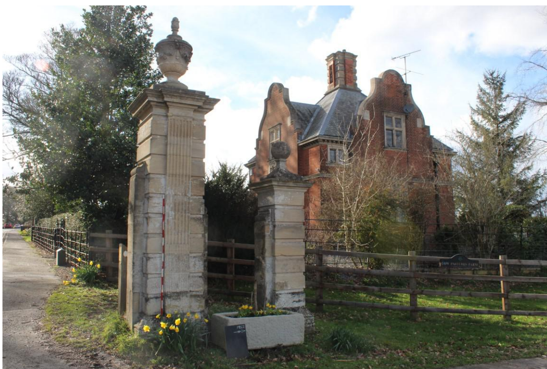
Plate 5: View of northern gate piers from southeast.
