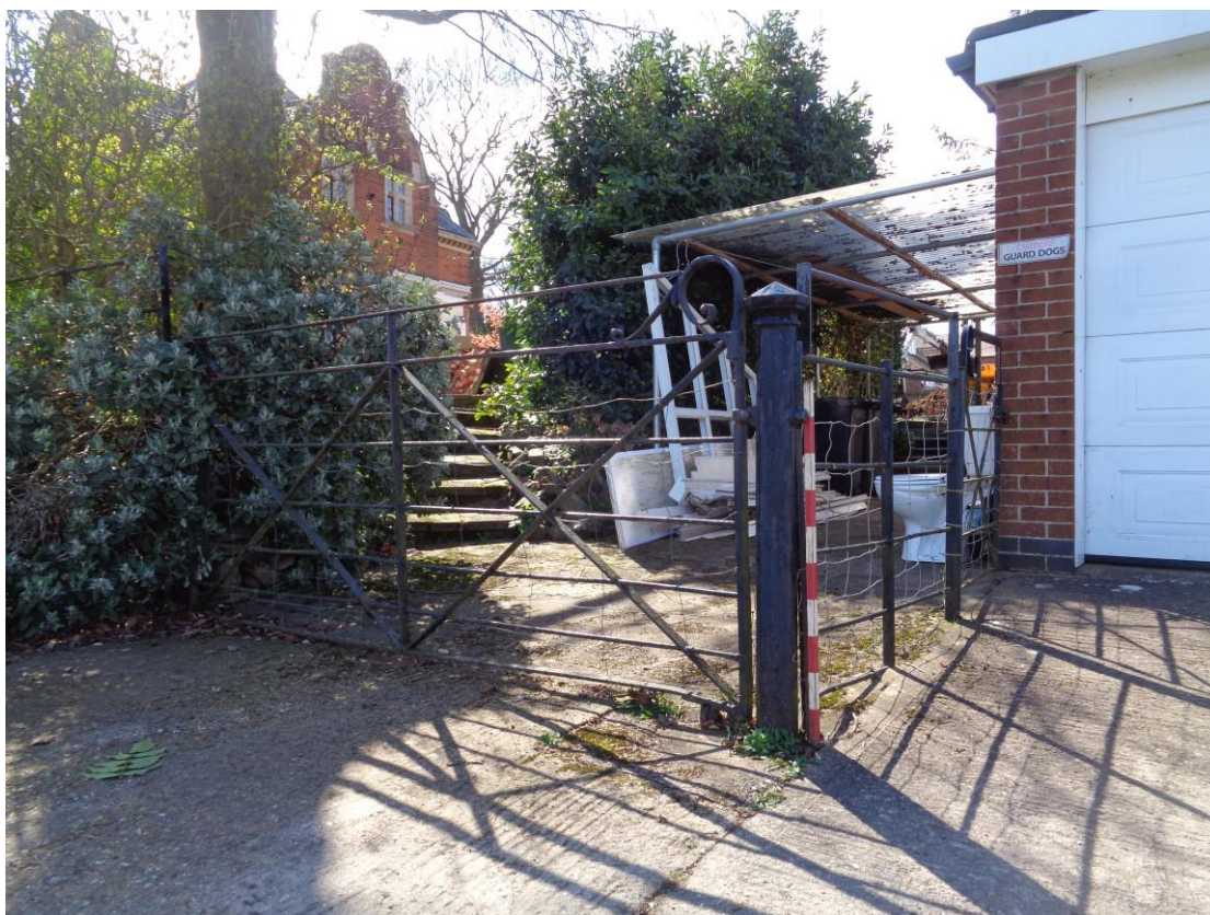
Plate 21: View of rear gates from northeast.
