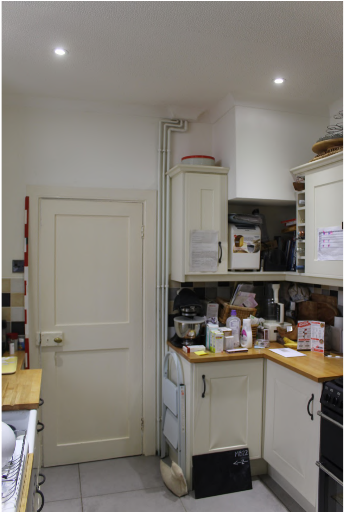
Plate 17: The kitchen showing an original utilitarian door and what appears to be the remains of a chimney flue over the site of a probable range.
