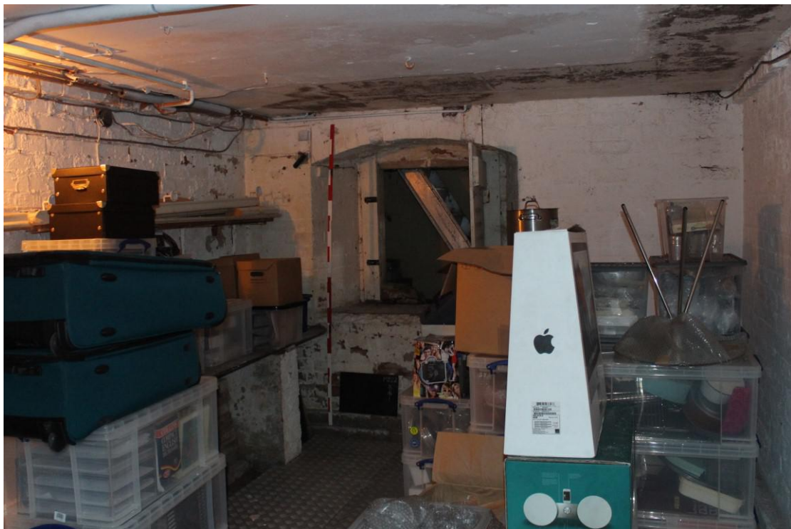
Plate 20: The cellar, showing the slate cold-shelf and the masonry of the casement window. The mullion was removed, a simple doorway added, and a short ladder inserted into the lightwell to provide external access.
