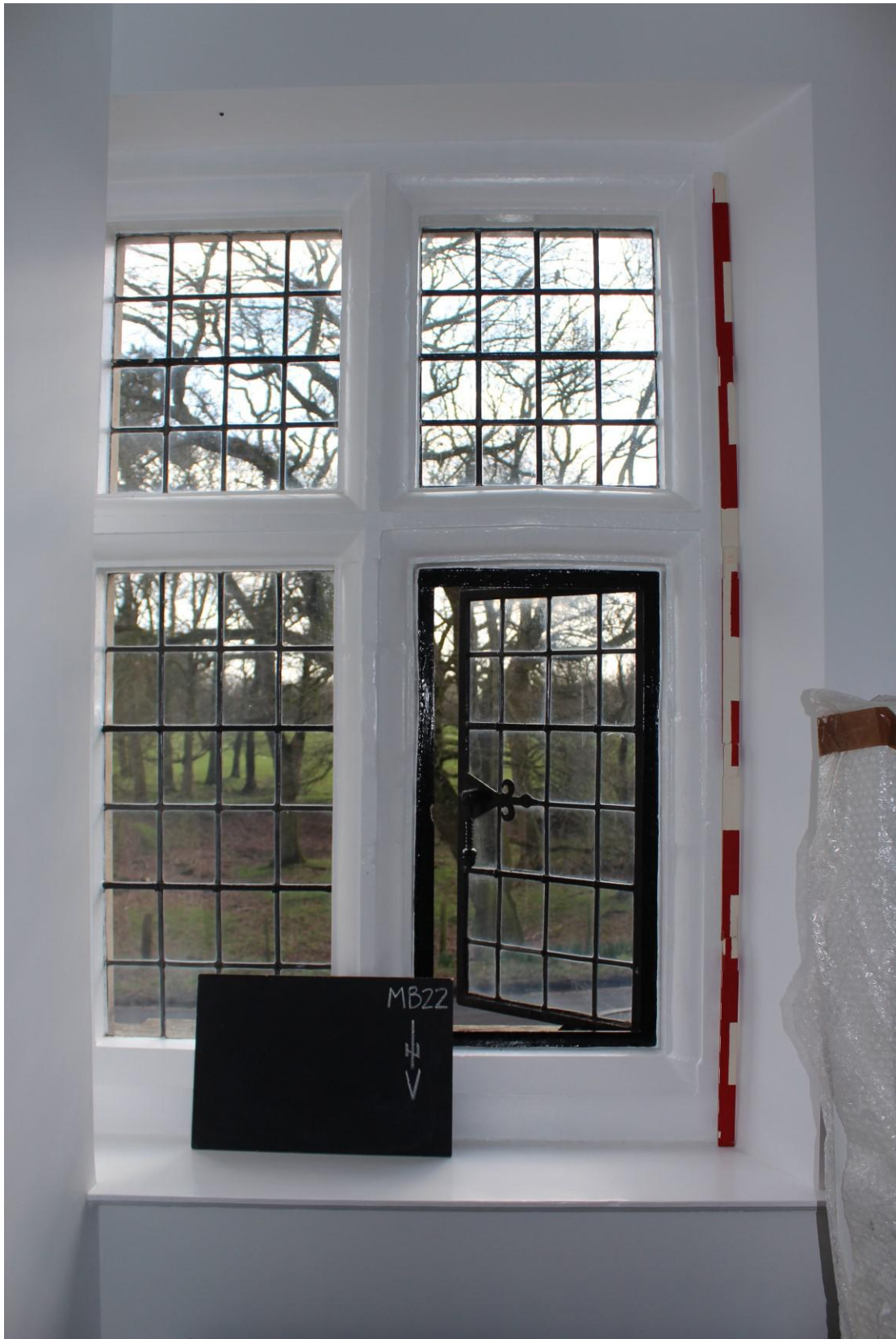
Plate 8: A 1st floor at the front partially blocked by an internal wall but preserving the symmetry of the front elevation.
