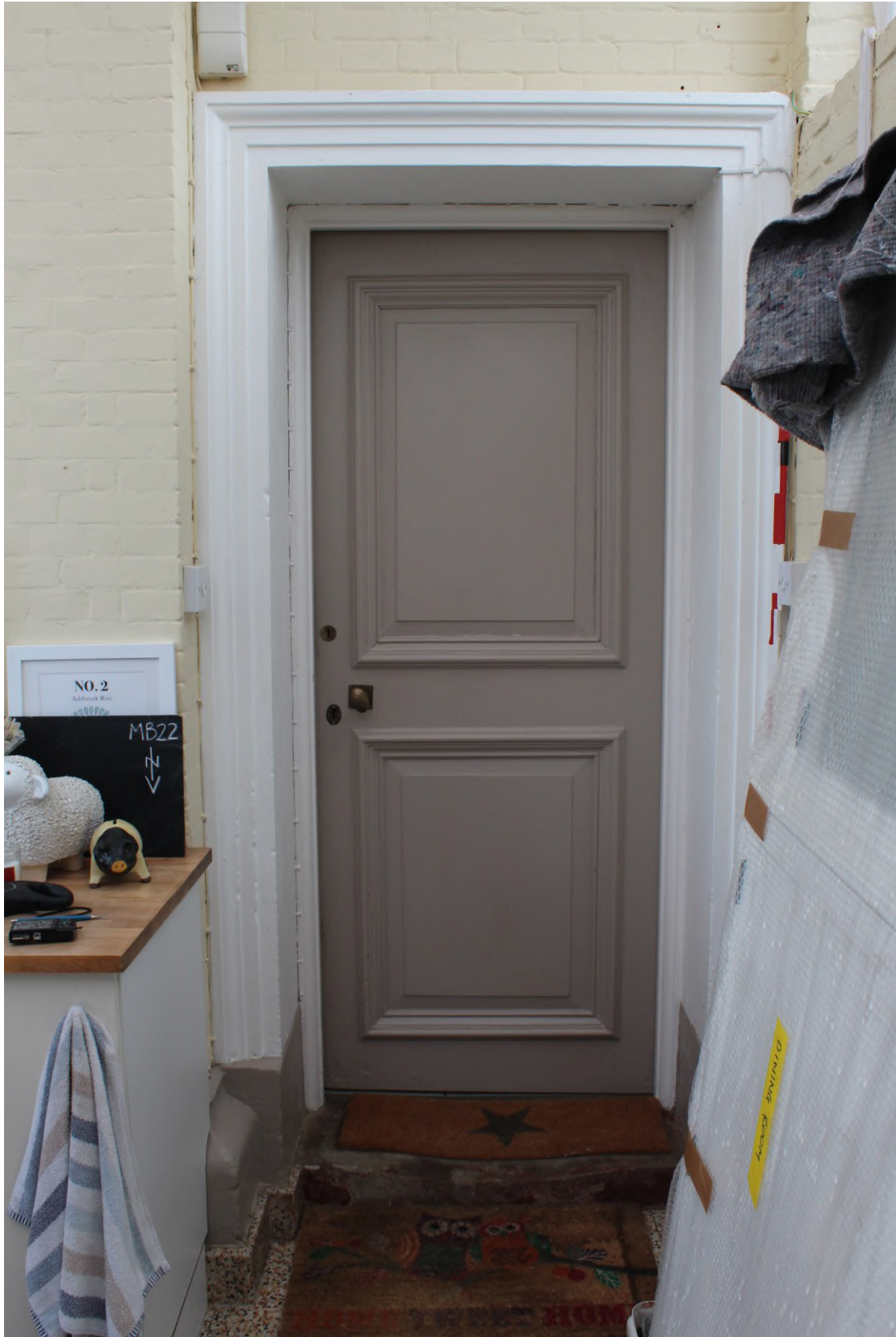
Plate 18: The former backdoor, note the worn step. The part of the original kitchen-yard here was roofed over and incorporated the old WC in modern times to provide a laundry and utility room. The doorway from the yard to the garden beyond was retained in the scheme as the existing backdoor.
