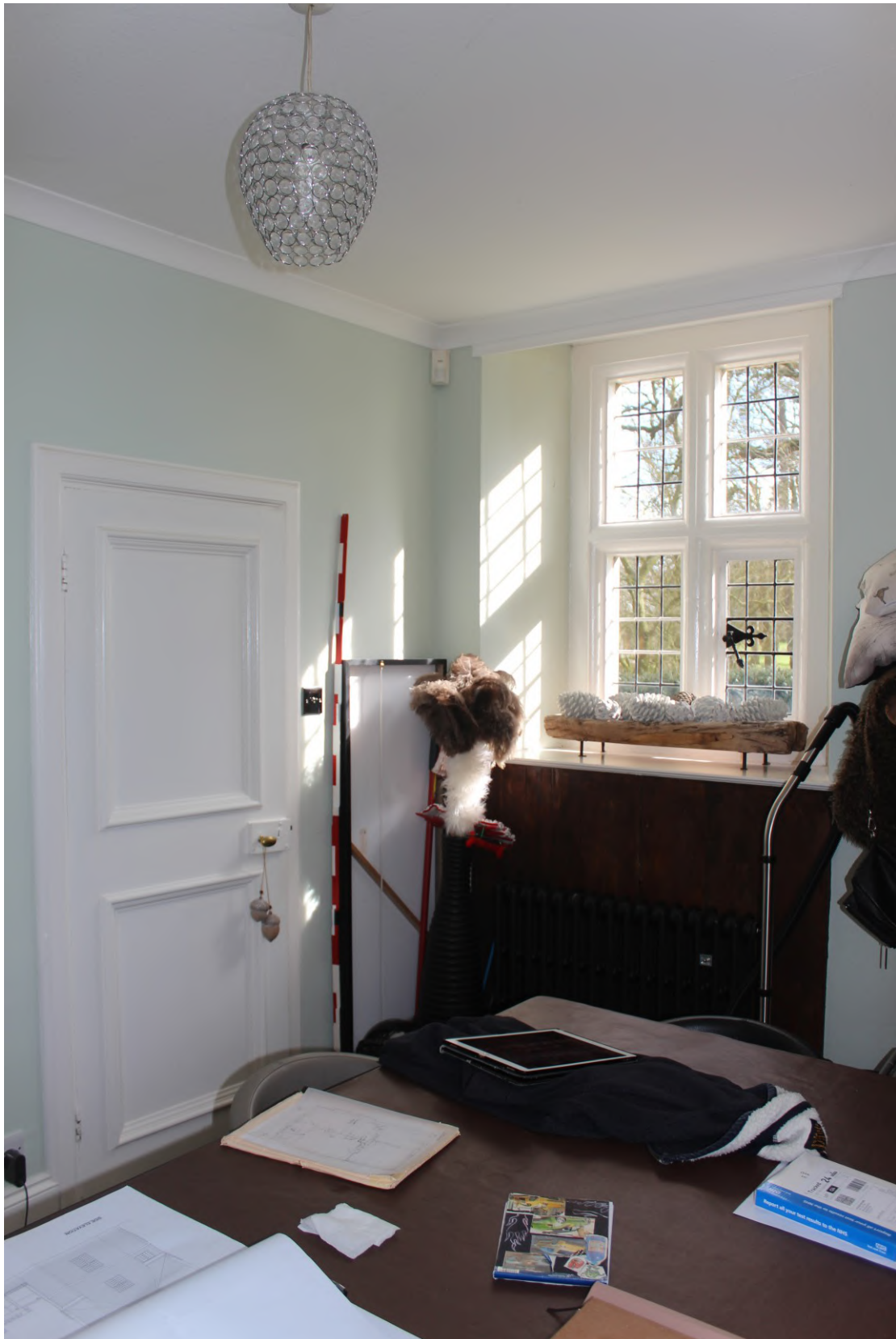
Plate 15: The dining room, showing a heavily moulded two-panel door, contrasting with the utilitarian doors on the 1st floor.
