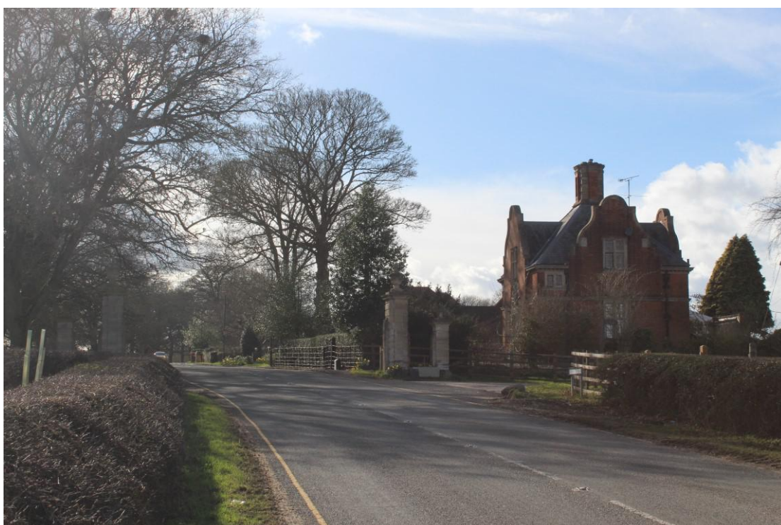
Plate 22: view from east showing present location of gate-piers. Compare this with fig. 11 view.
