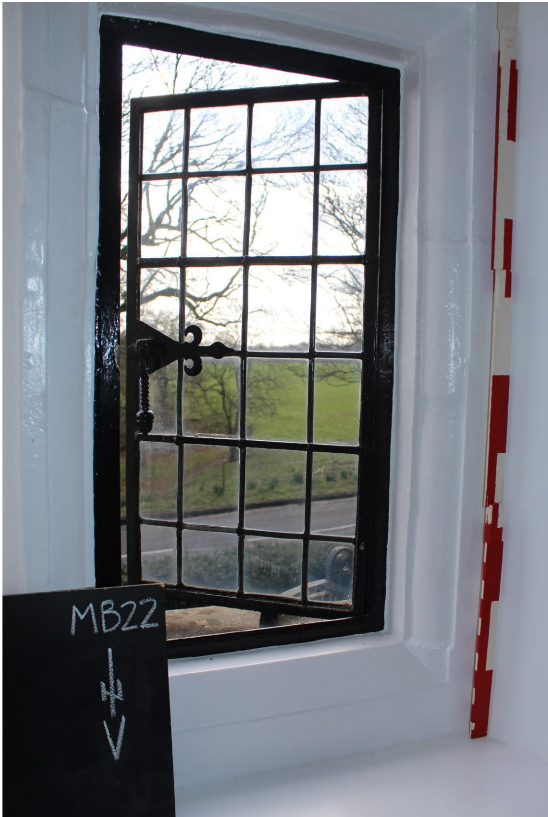
Plate 9: Detail of window's iron fittings and furnishings.
