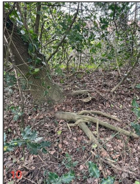
Picture 12. T10-Partially uprooted ash with minor basal movement when pushed by hand.
