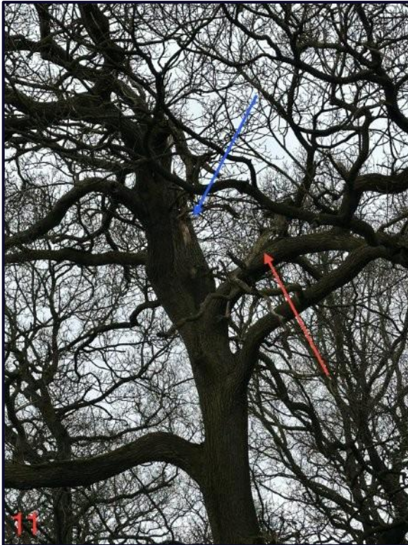
Picture 13. T11-Oak with snapped hanging branches indicated by red arrow and decayed central stem indicated by blue arrow.
