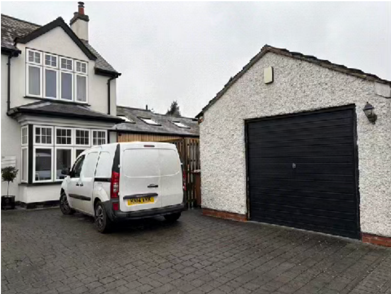
Existing large single storey garage looking rather sad against the renovated house.
