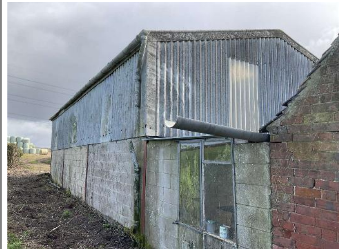
B1 - northern and western elevation
