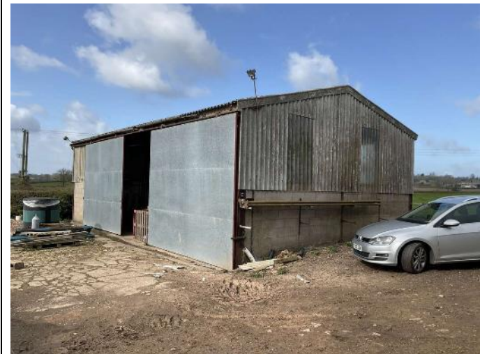
B1 - southern and eastern elevation
