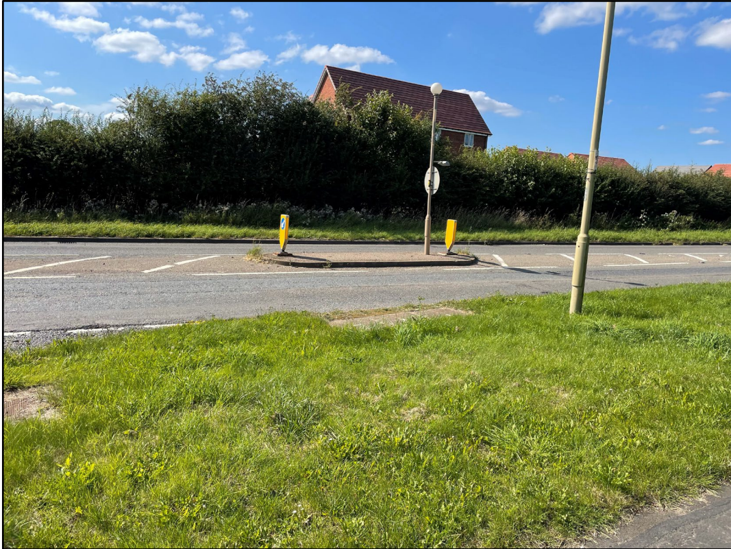
Figure TN6.3: Existing Traffic Island on Normandy Way North of Outlands Drive
