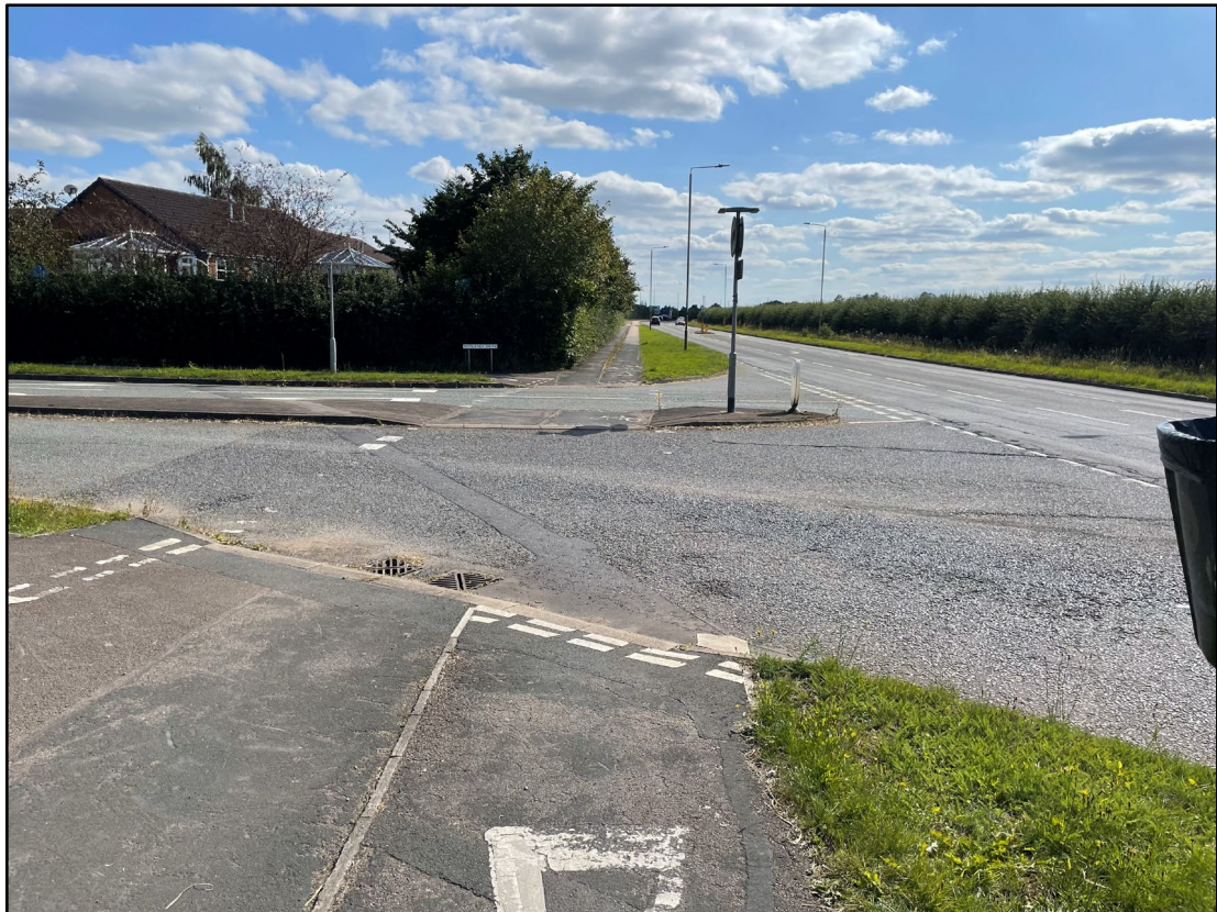
Figure TN6.2: Existing Pedestrian and Cycle Facilities at Normandy Way/Outlands Drive Junction (looking south)
