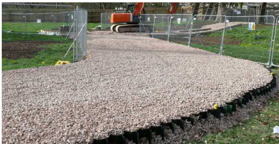
Figure 4 - Example of temporary Cellweb® construction solution
