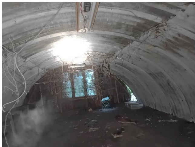
Photo 12: Internal of building B2b.
