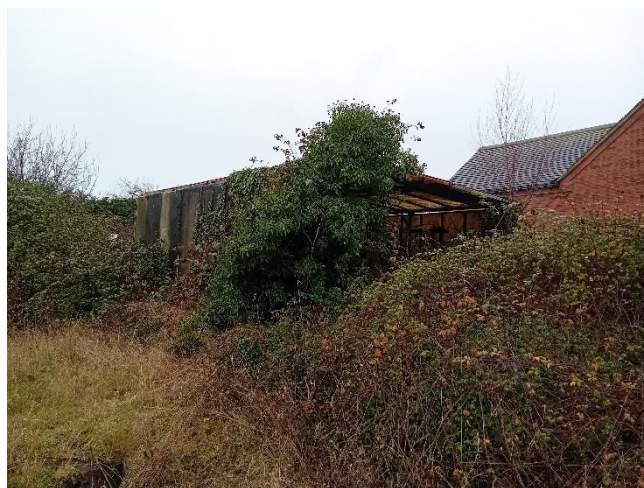
Photo 8: North and west elevations of building B2a.
