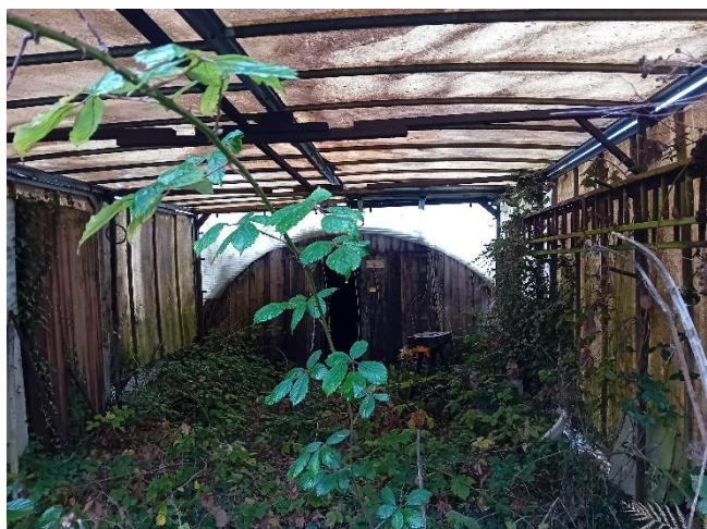
Photo 9: Internal of building B2a.
