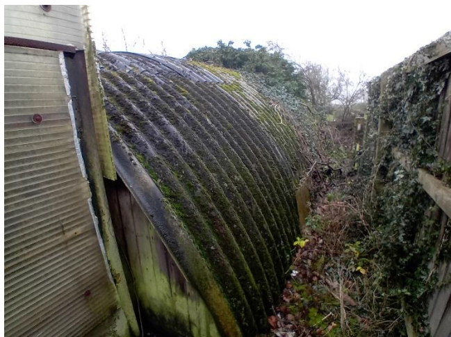
Photo 11: North and west elevations of building B2b.
