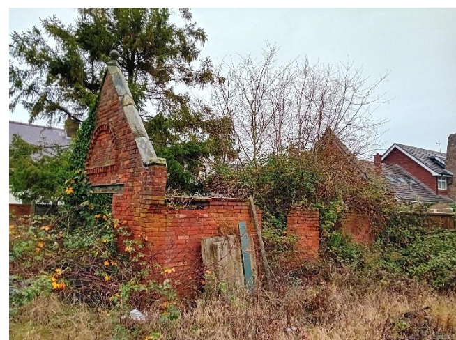
Photo 5: South and west elevations of building B1.
