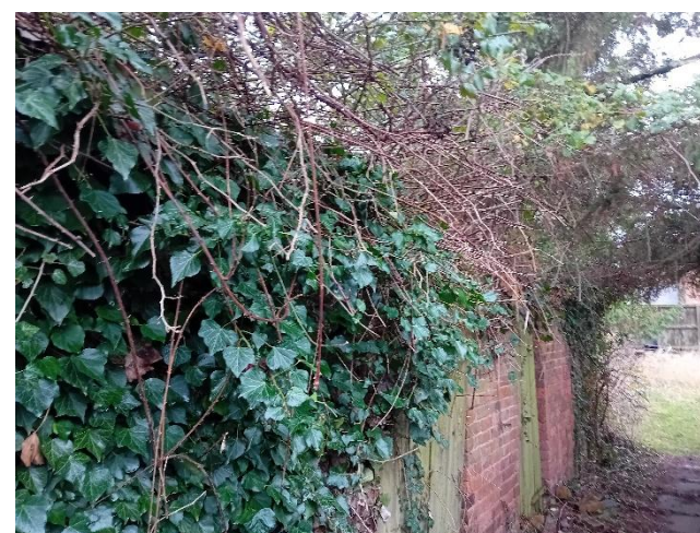
Photo 6: North elevation of building B1.
