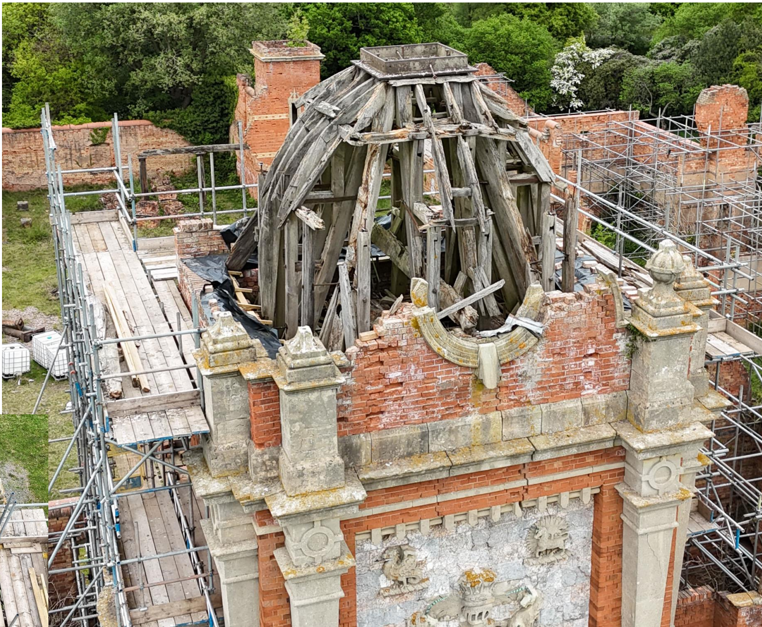
View of Timber Cupola to be Dismantled and Set Aside for Reuse
