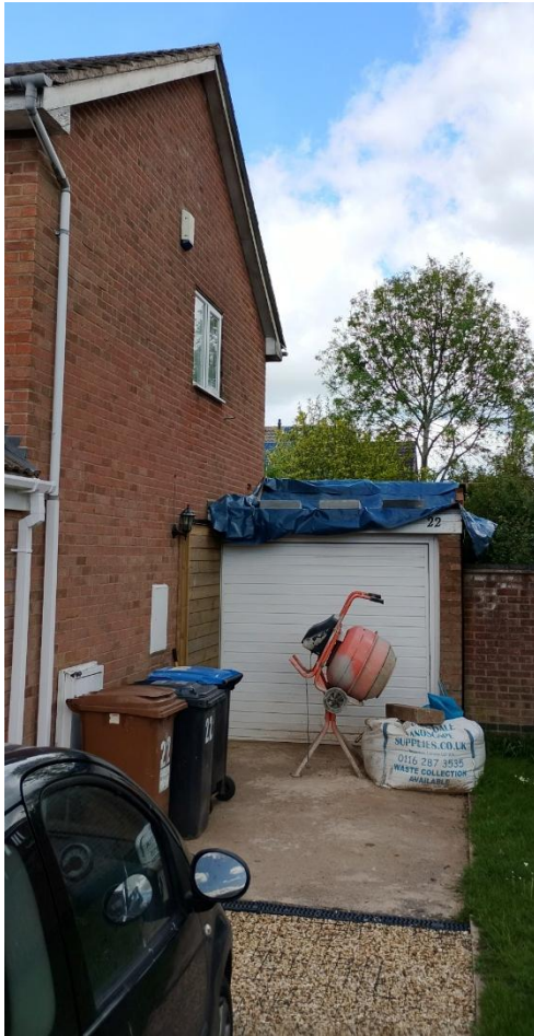
Figure 1: Side elevation of the surveyed building and attached garage structure.
