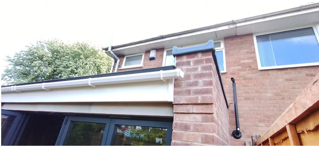
Figure 6: Rear elevation and extension roofline showing external features.
