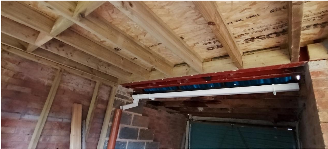
Figure 5: Internal view of garage roof structure and extension works.
