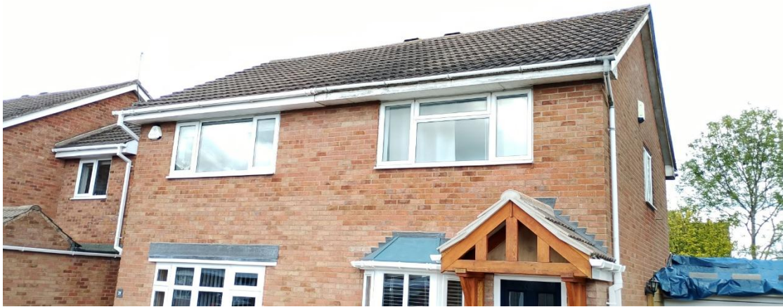
Figure 7: Front elevation of the surveyed dwelling.
