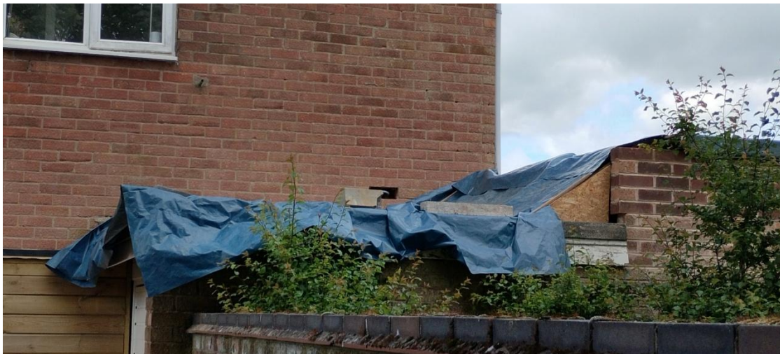
Figure 10: Detached garage structure and adjacent vegetation within the rear garden.
