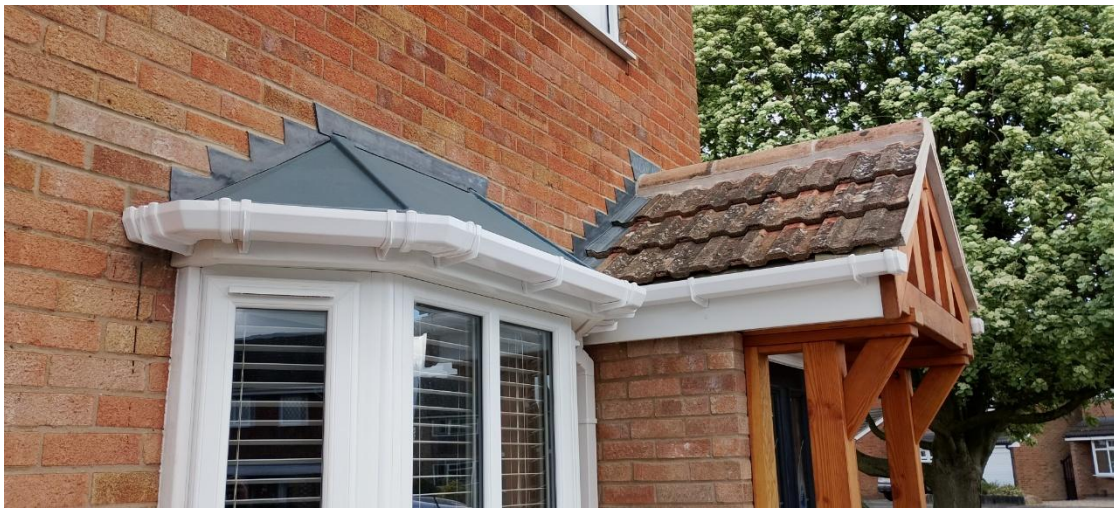
Figure 8: Front porch and roof junction detail.
