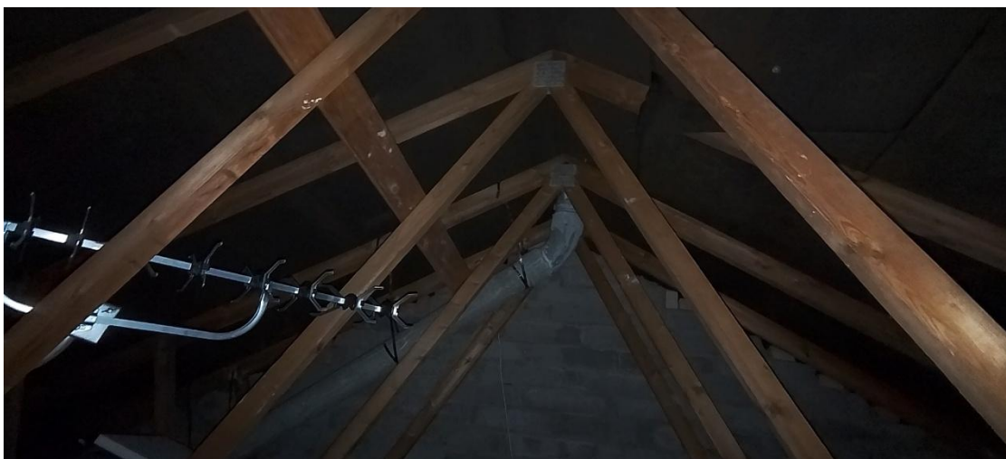
Figure 2: Internal loft void showing exposed roof timbers and internal roof structure.
