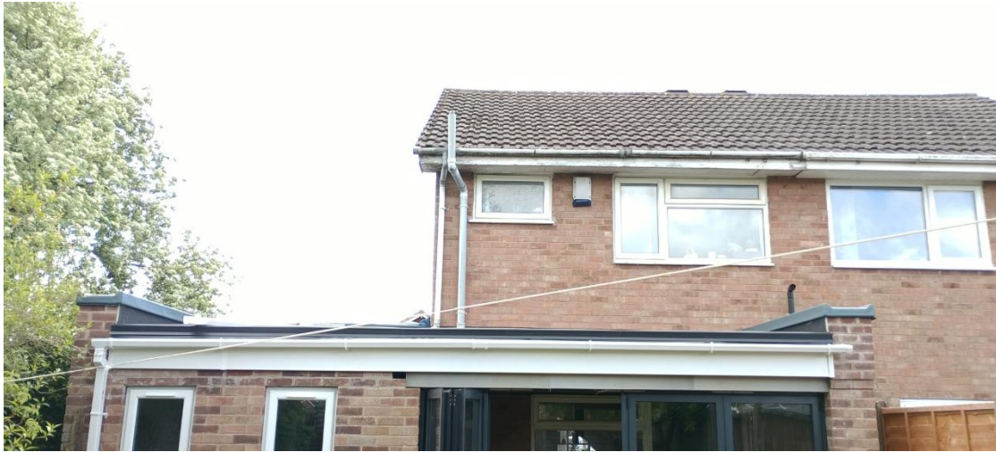
Figure 3: Rear elevation of the surveyed building and single-storey extension.
