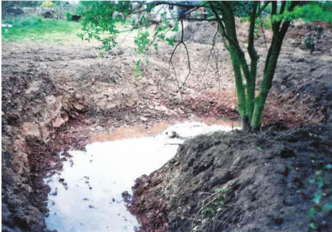
(b) Taken 2006 (shows construction of the northmost pond)
