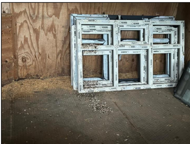
Photograph 16: Bird droppings in B2
