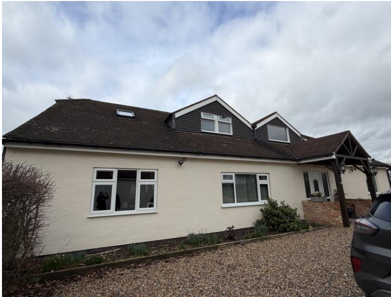
Photo 1: The existing residential building that will be extended and modernised within the proposed development.
