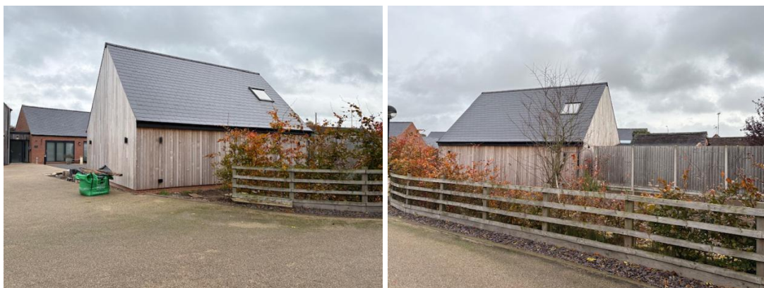
Figure 10 - Exposed nature of adjacent garage
