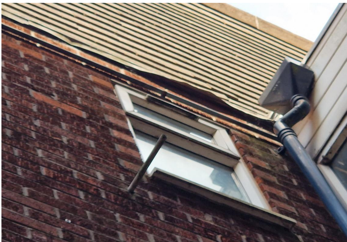
Plate 10: Image showing the lifted flashing on the southern elevation of B1 .
