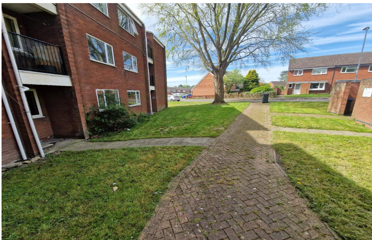
Plate 6: Image showing the northern elevation of B2 .
