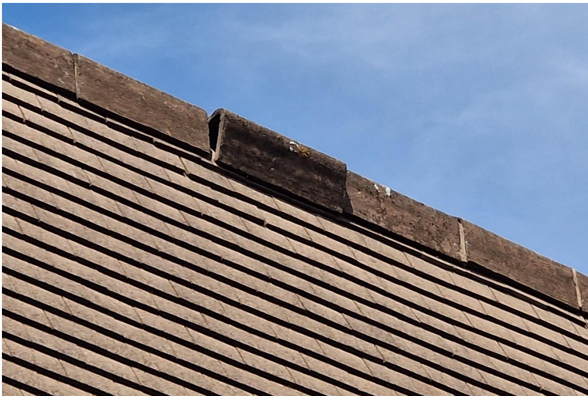
Plate 14: image showing the ridge vent on B1 .
