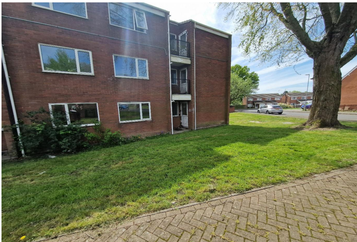
Plate 5: Image showing the northern elevation of B2 .
