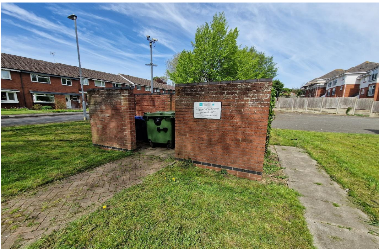
Plate 24: Image showing the wall on the centre of the site.
