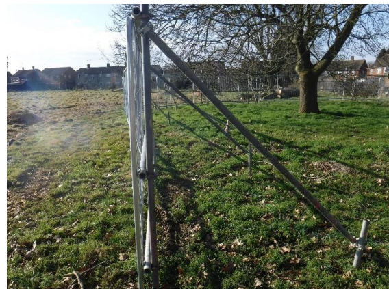
Photo 6: Scaffold driven into ground
