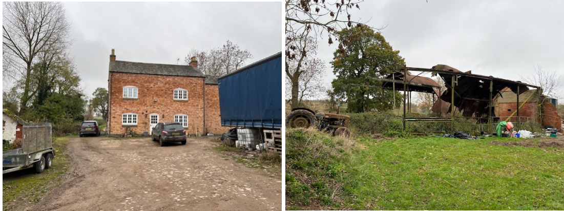
Figure 4 - Photograph showing existing trailer and partially demolished dutch barn
