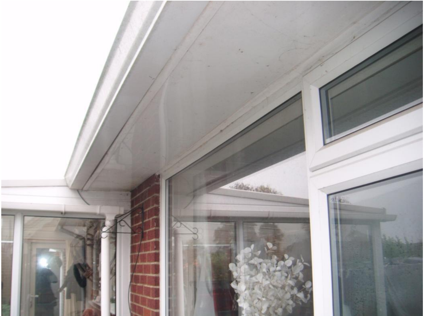
Rear soffits and conservatory
