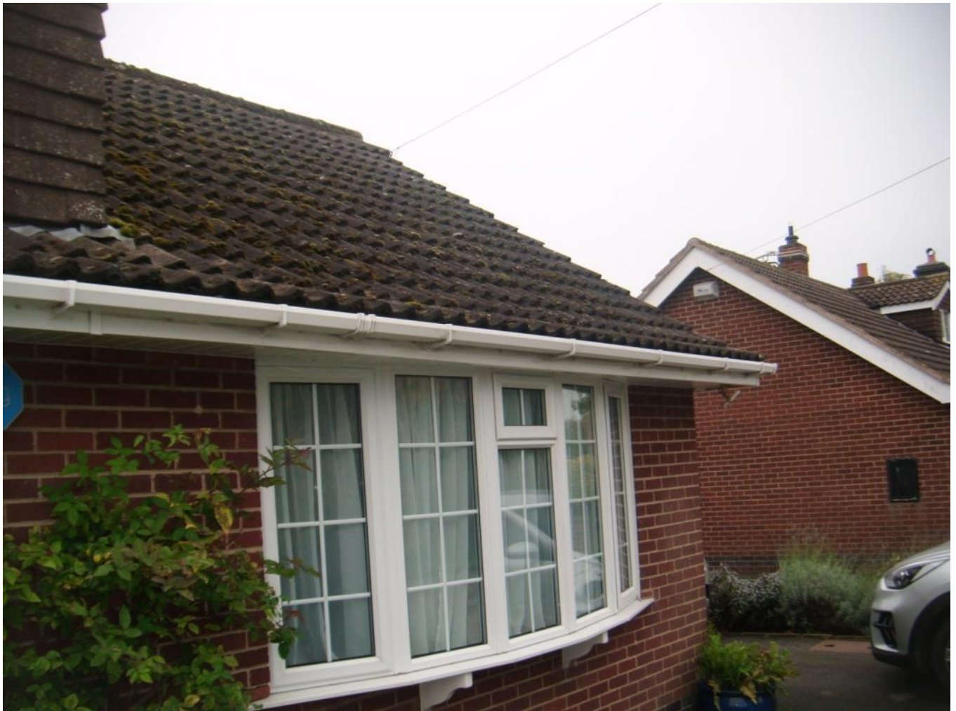
Front soffits/roof intact
