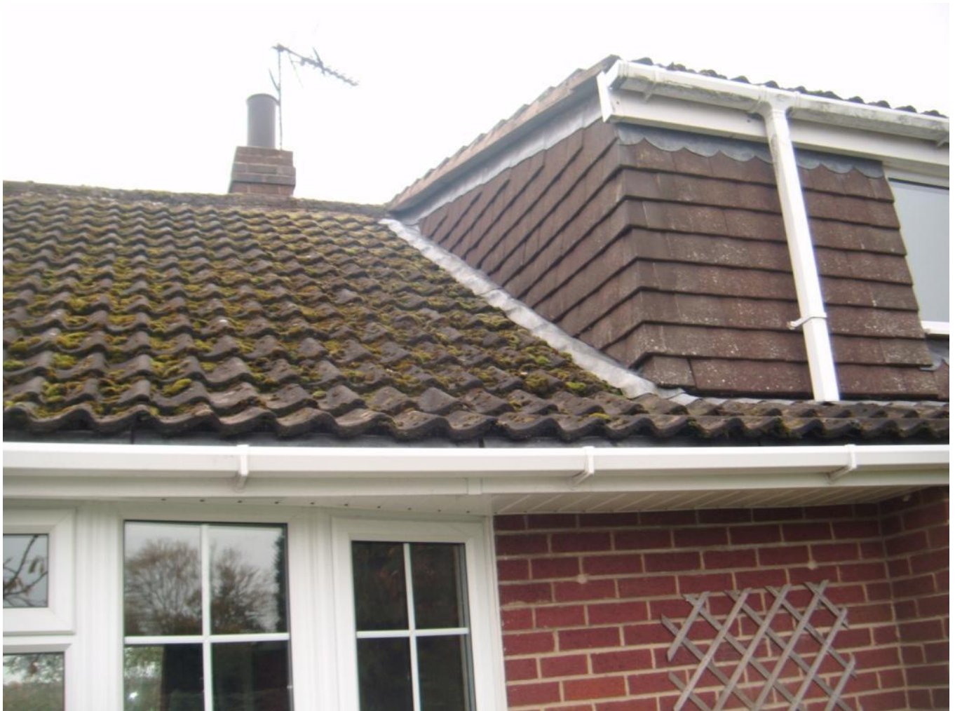
Intact front dormer
