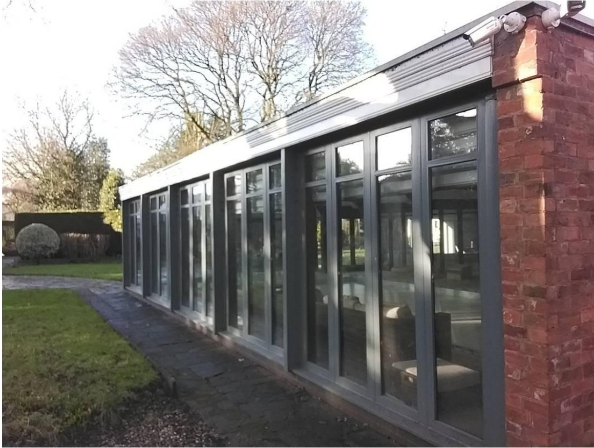
Photo 2. Existing residential building (B4) in the south unaffected by current proposals
