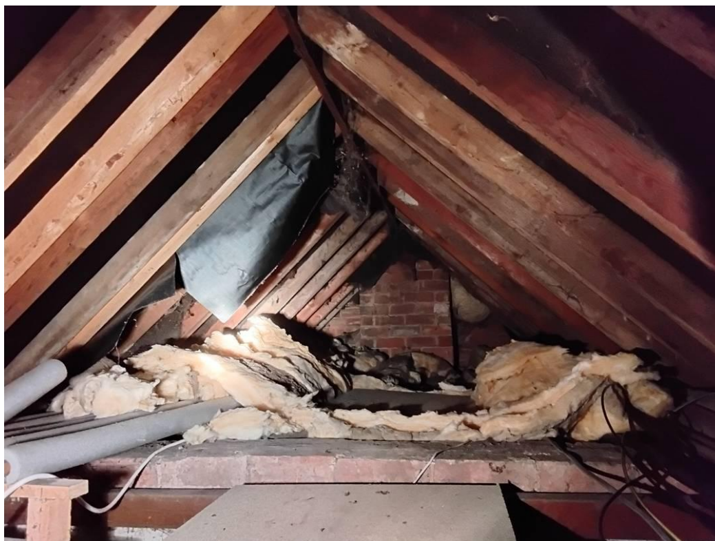
Photo 13. Crawl space of B1, with chimney at the rear.
