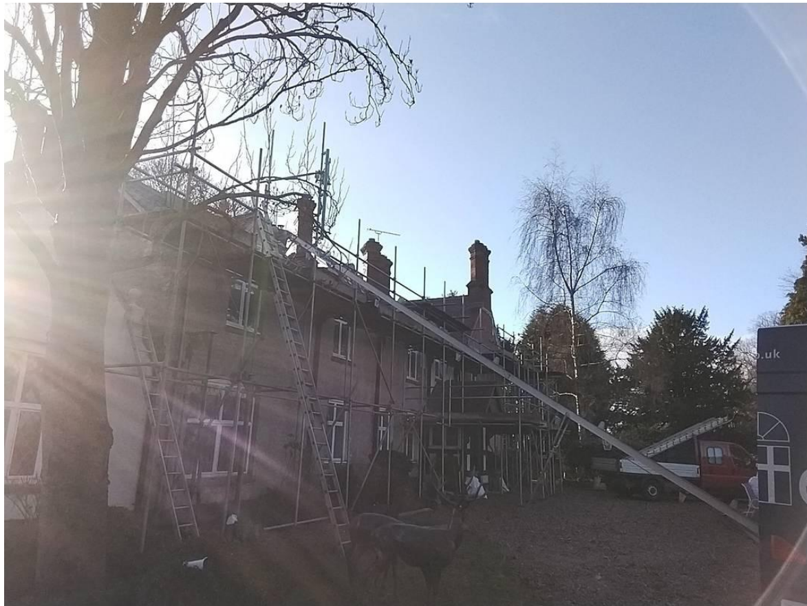
Photo 1. Existing residential building (B3) which is unaffected by current proposals
