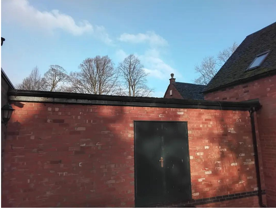
Photo 16. B2, constructed of brick with a flat roof
