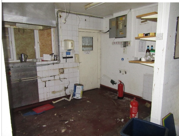
Former Commercial Kitchen
