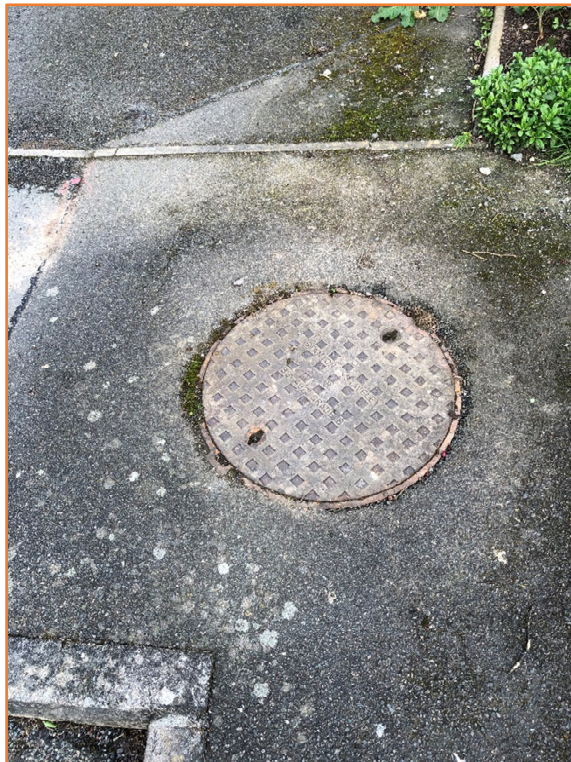
Photo of manhole 3703 within Beech Drive, which is a continuation of the existing Severn Trent surface water sewer.
