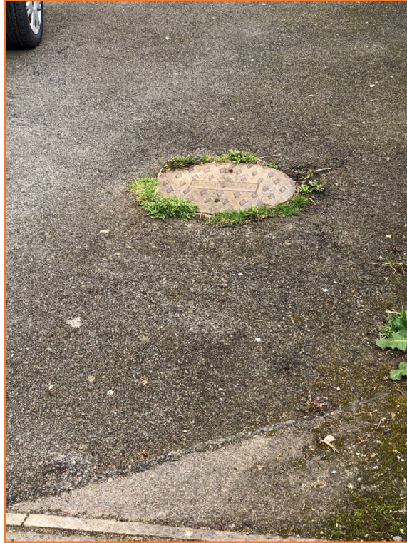
Photo of manhole 3702 within Beech Drive, which forms the head of the existing Severn Trent foul sewer.
