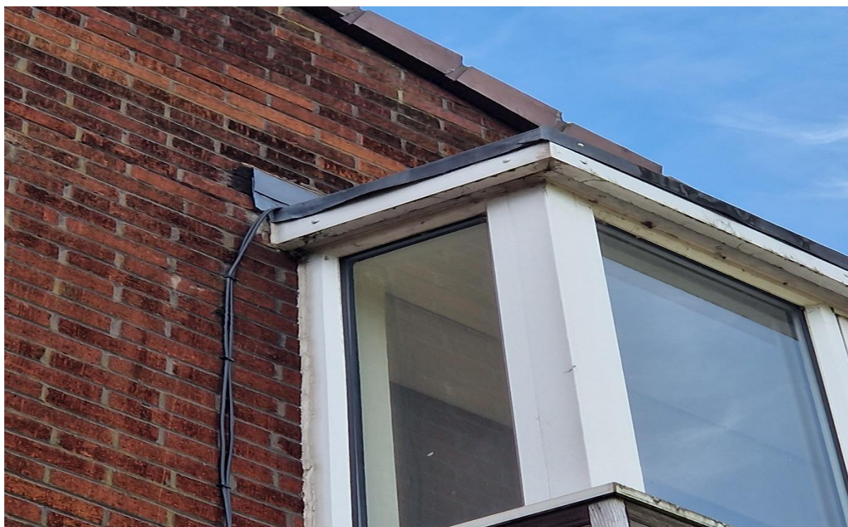
Plate 11: Image showing the drip edge vent on B1 .
