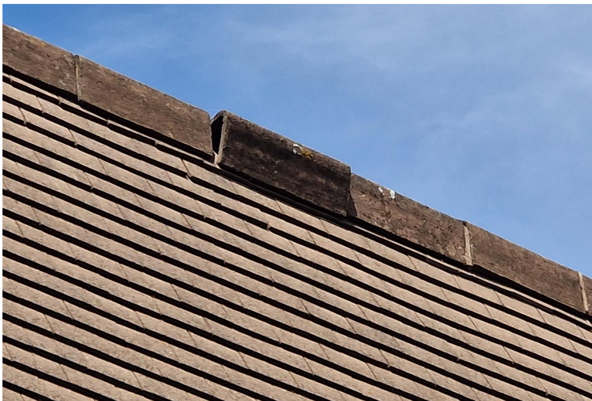
Plate 14: image showing the ridge vent on B1 .
