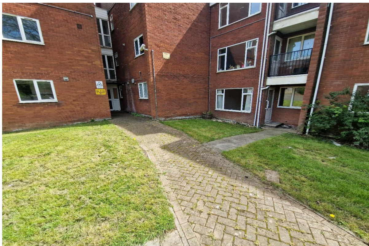
Plate 7: Image showing the western and northern elevation of B1 and B2 .
