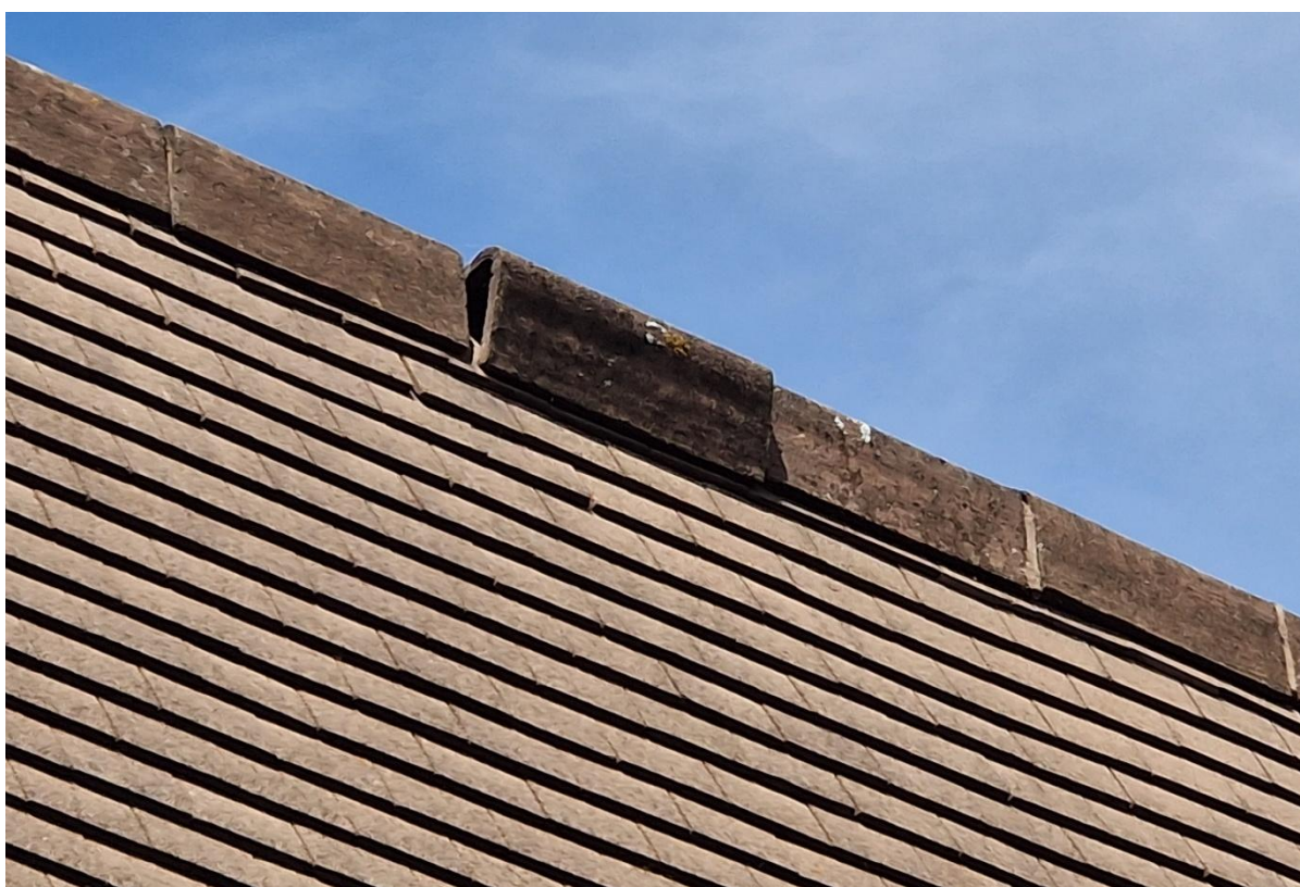
Plate 14: image showing the ridge vent on B1 .
