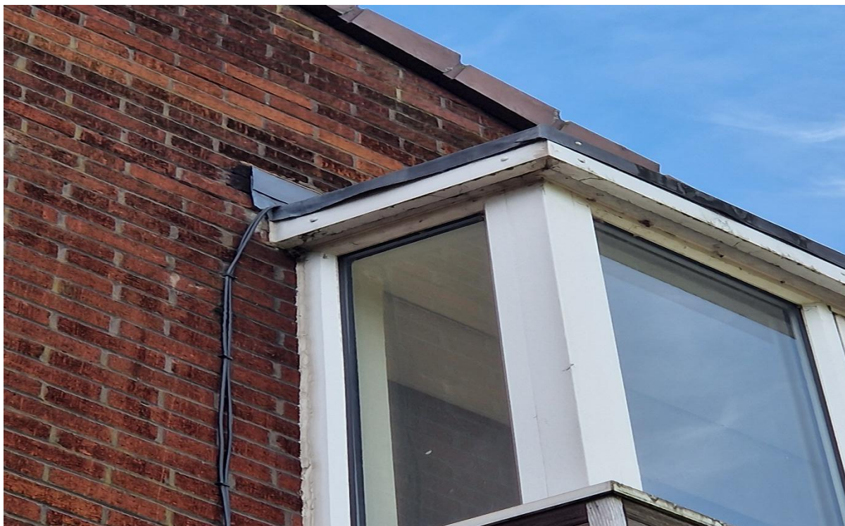
Plate 4: Image showing the lifted flashing on the southern elevation of B1 .
