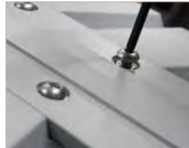
Step 6 Mount new LED chevron to the luminaire spine
