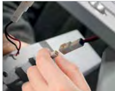
Step 5 Plug in new LED chevron using existing 'plug & play' connectors on the luminaire spine
