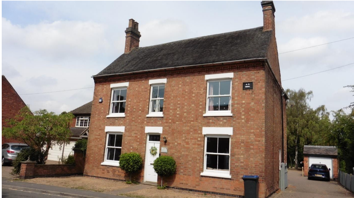
Photograph 1: the frontage to 39 Main Street, Carlton. This shows the two-storey traditional dwelling section being retained as part of the development.
