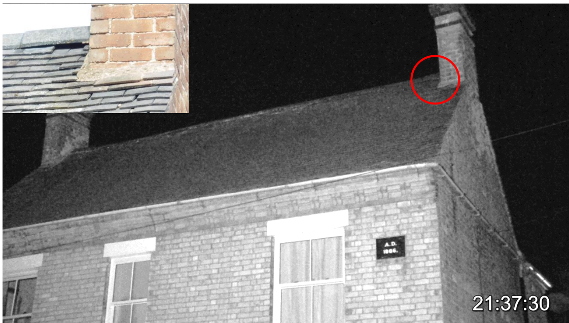
Figure 2 - Field of view from Camera F at end of survey 21:37:30. The bat emerged from the area encircled in red.
