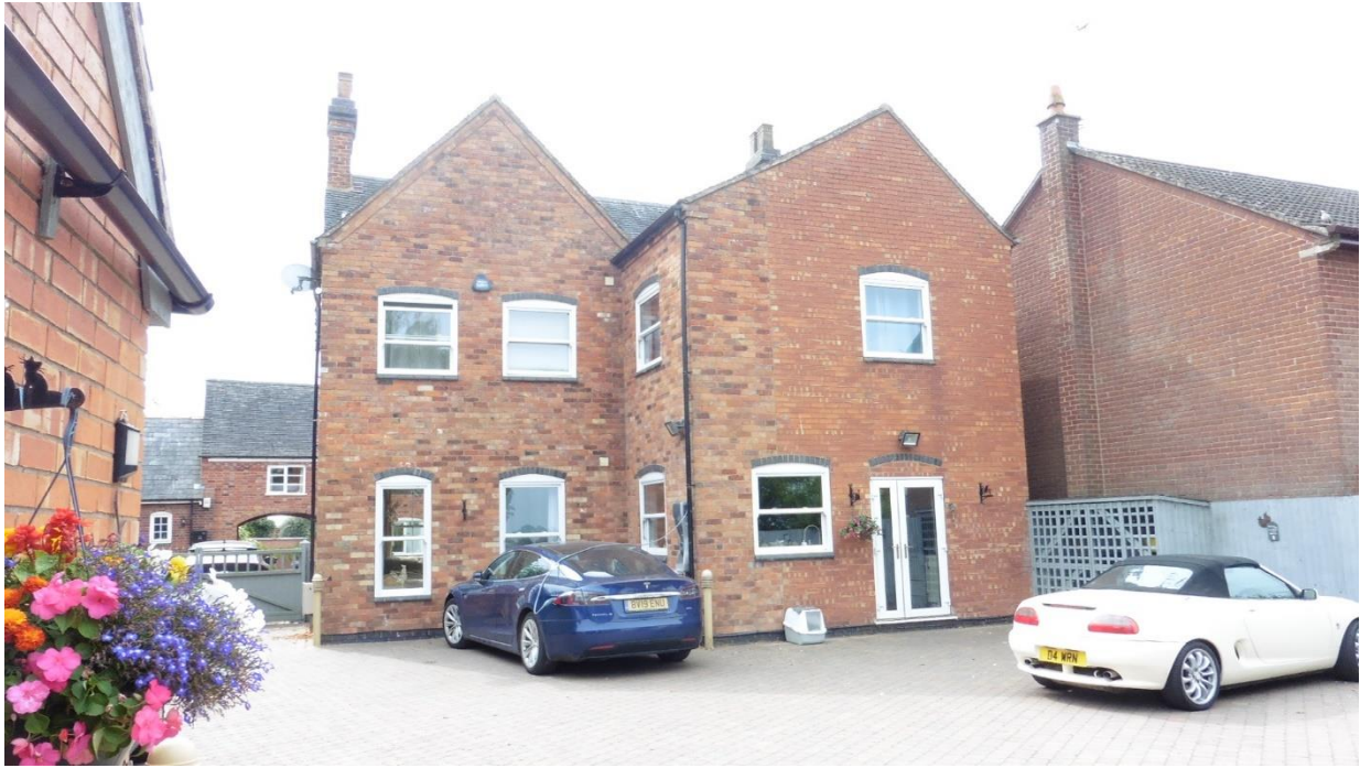
Photograph 3: showing the two house extensions proposed for removal to make way for the redevelopment.
