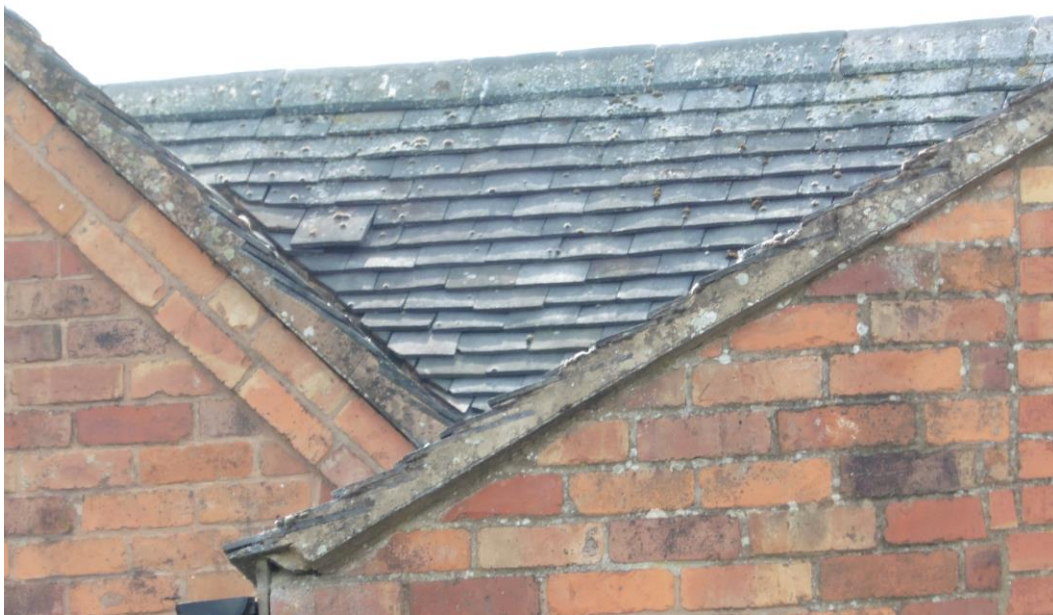
Photograph 9: example of the multiple gaps present under the existing rosemary tiles on the traditional house section.
